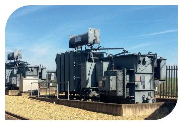
Figure 19: Two 33/11kV primary substation transformers during a visit to a LEAN project trial site
