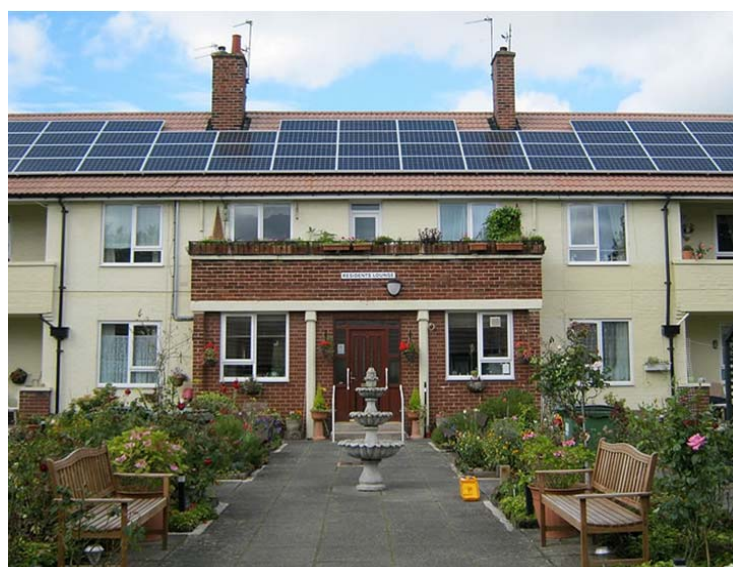
Figure 2.3: PV installed on sheltered accommodation by Stockport housing
