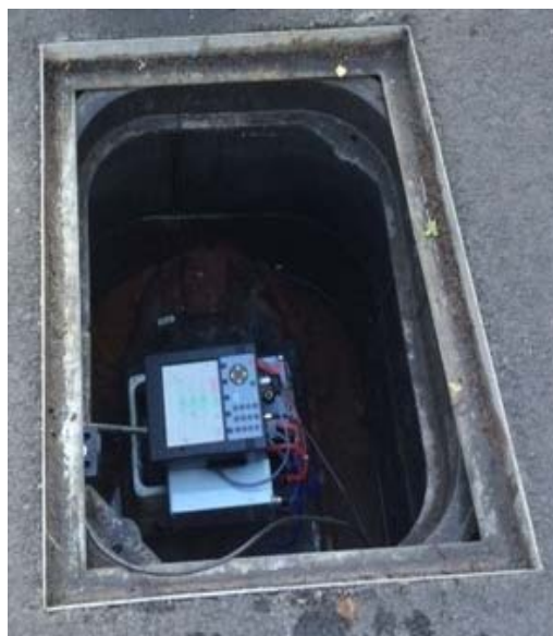
Figure 2.10: LV switches installed in a link box
