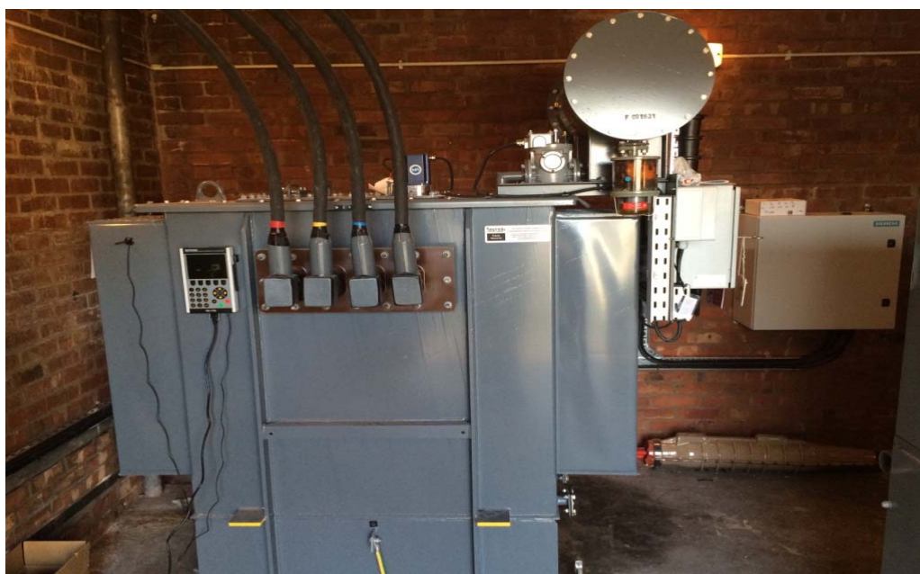
Figure 2.8: Distribution transformer with OLTC
