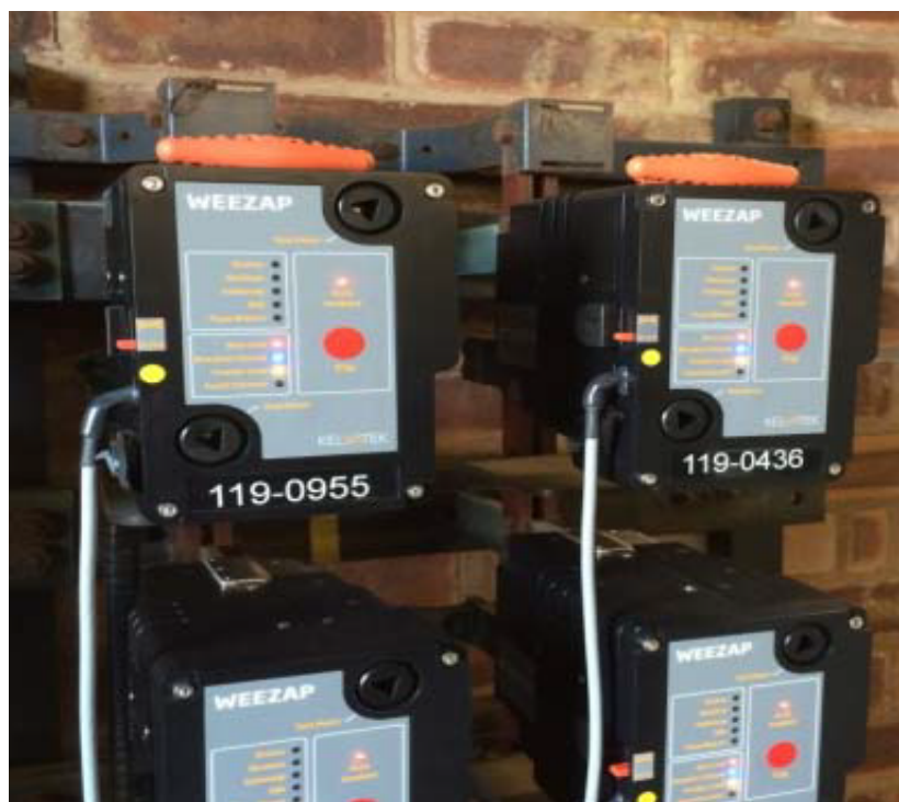
Figure 2.9: LVCBs installed in a distribution substation
