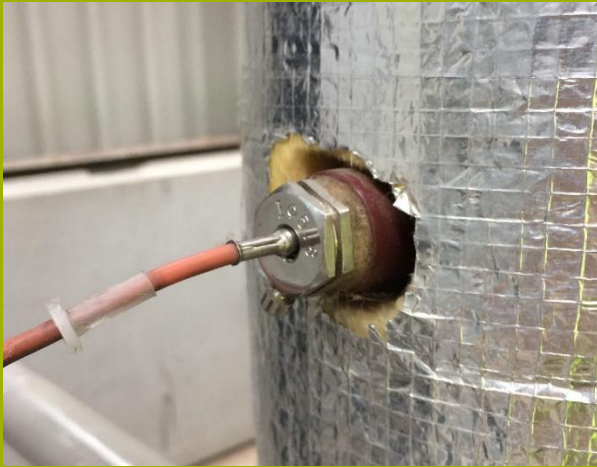
1. The sensor is installed incorrectly. Also a security tag should be attached
