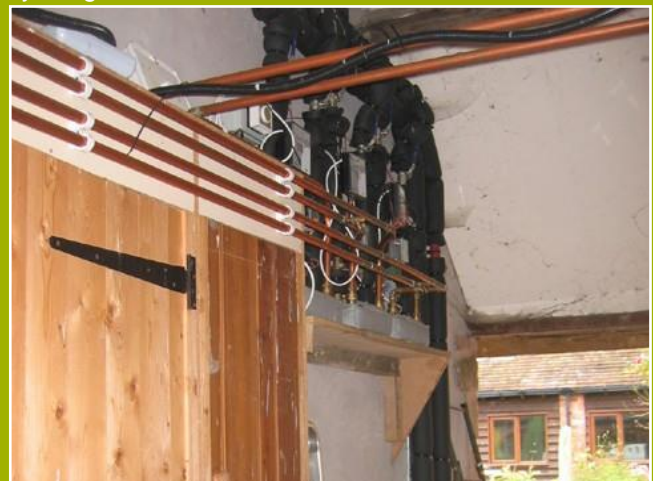
4. The pipework was wrongly declared as internal. It is external pipework as it is in an open corridor.
