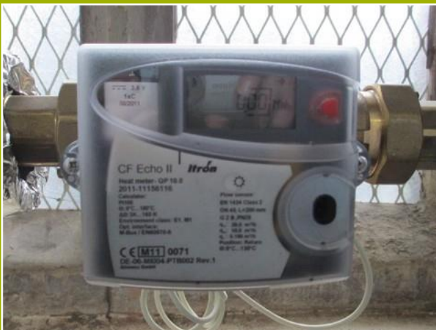
3. The probes on the meter have not been connected and so there is a zero meter reading.
