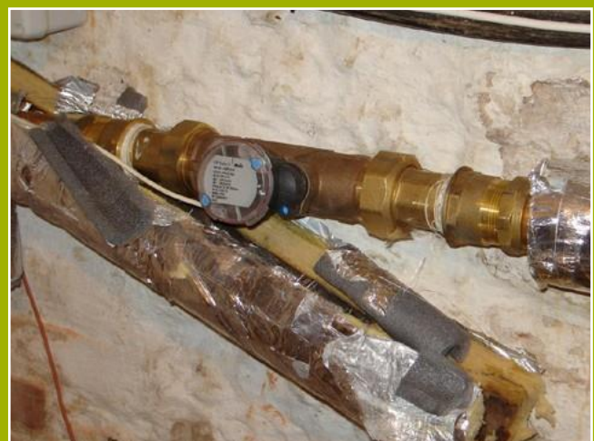
6. 'After' photo shows correct meter orientation
