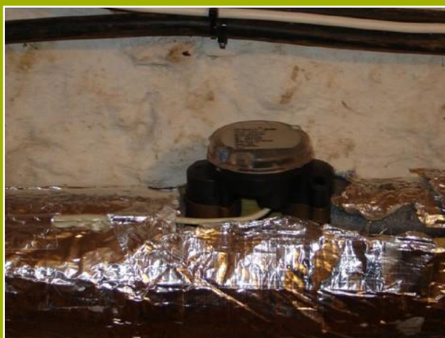
5. 'Before' photo shows incorrect meter orientation
