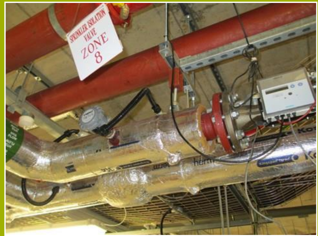
2. The meter is in the flow pipe rather than the return pipe. The flow pipe is clearly identified as seen by the green label and the witness mark arrow.
