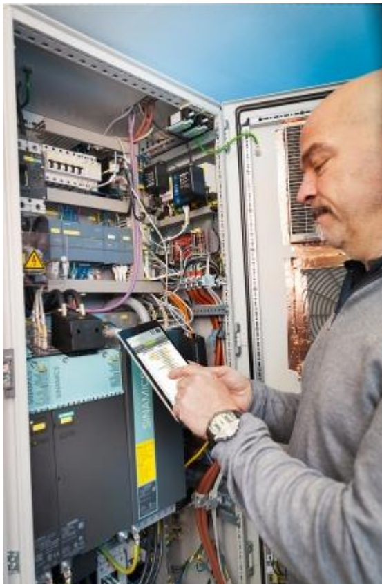
Cabinet with lithium-ion batteries and electronic switchgears
