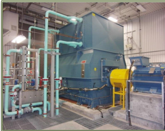
Figure 41 ABB Synchronous Compensator
