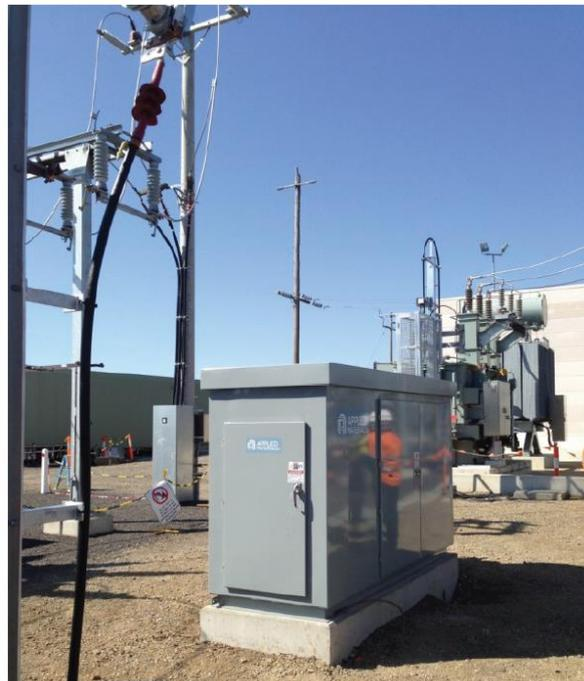
Figure 17 - SSFCL installed in Australia
