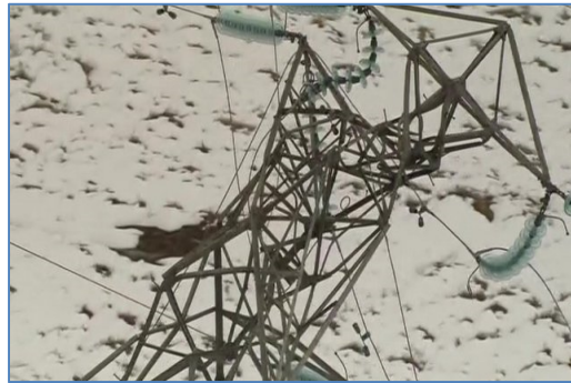
Figure 2.3: Steel lattice tower in construction Figure 2.4: Fallen tower after 2013 snow storm
