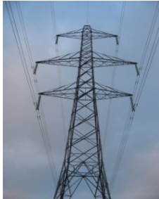
Figure 2.2 Traditional steel lattice suspension supports
