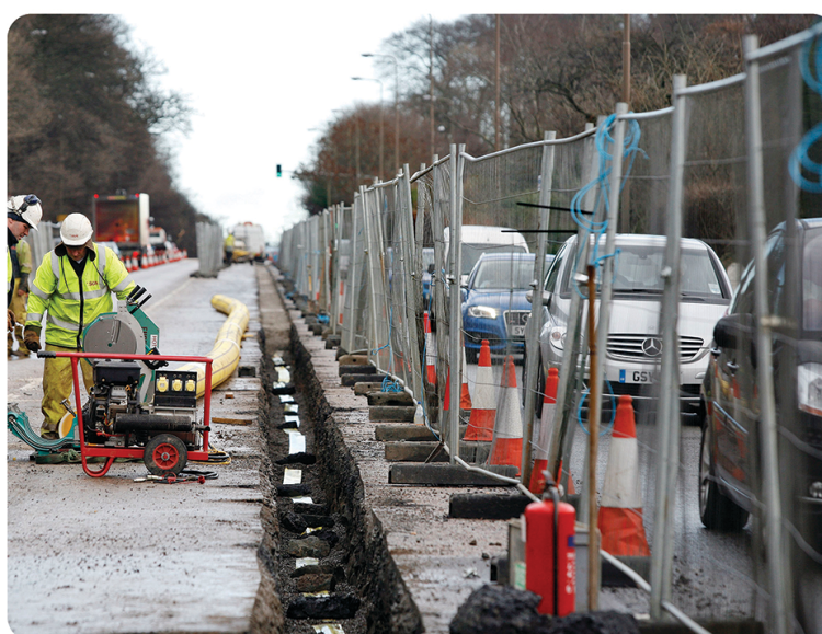
Fig 10.1: Open-cut mains replacement siteworks
