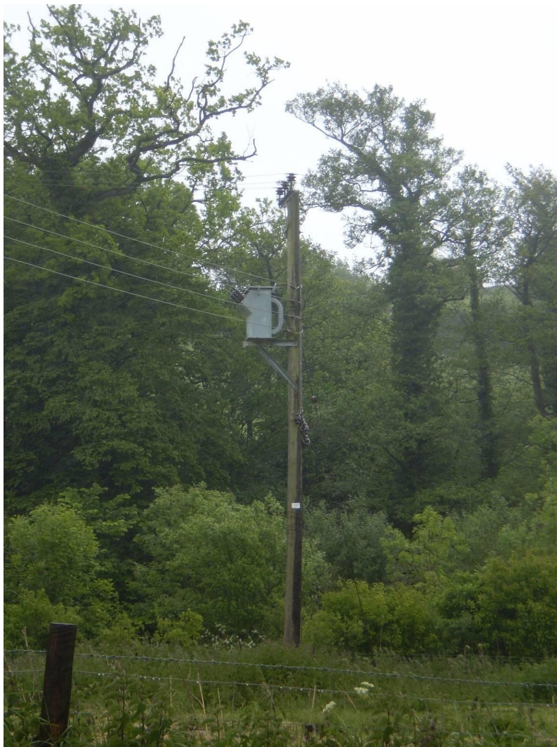
Pole Mounted Transformer (PMT) – 11kV
