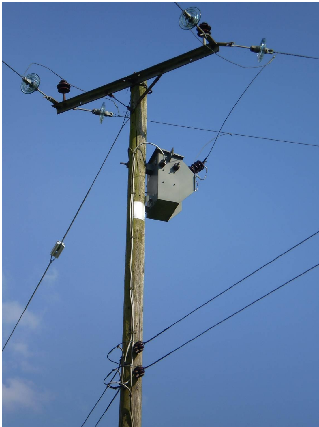
Pole Mounted Transformer (PMT) – 11kV
