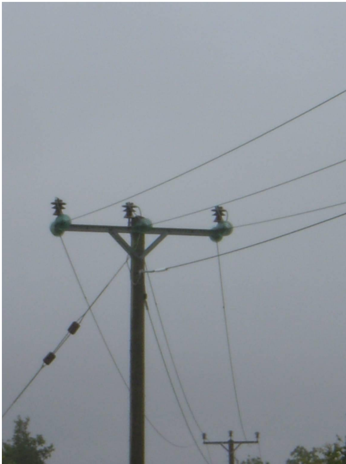
Intermediate Pole (upright pin type insulators) – 33kV shown here
