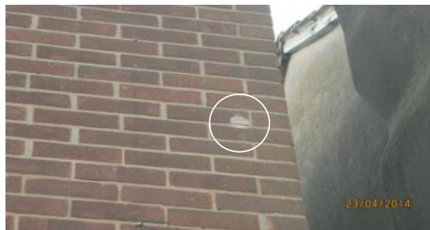
Figure 3 – Evidence of drill hole used for lance installation of CWI
