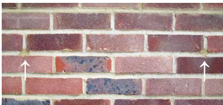
Figure 6: Position and size of standard drill hole
