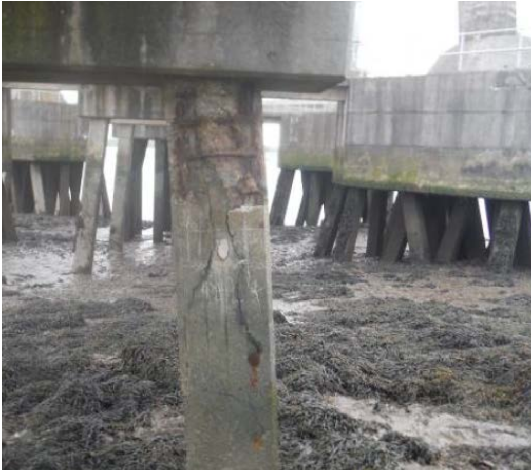
Figure 24: piled foundation XD130. Rebar exposed.
