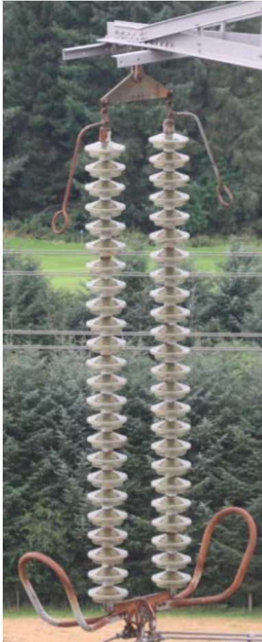
Figure 25: rust degraded suspension insulator set at ZC(N) Route.
