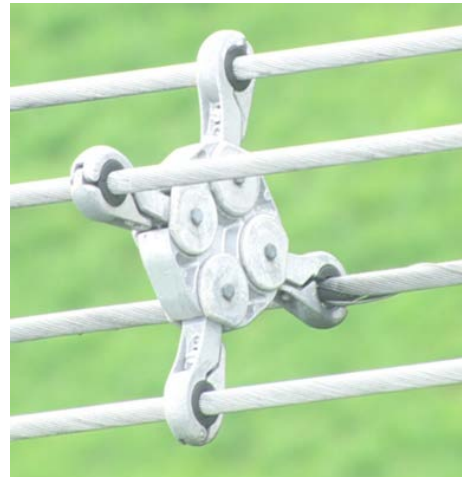
Figure 8: conductor damaged at 'Dunlop' spacer-damper clamping position at ZP Route (062-063).
