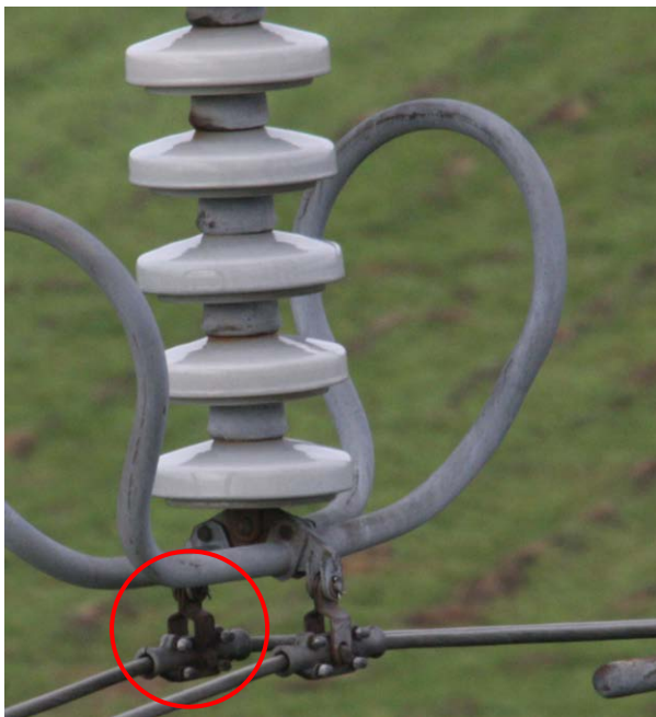
Figure 18: level of rust at ZE Route porcelain insulator caps and wear of suspension strand.
