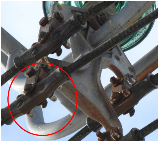
Figure 11: worn suspension strand and cotter pin at ZP Route
