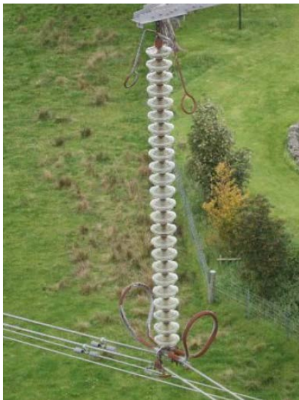
Figure 21: suspension set at ZF Route.
