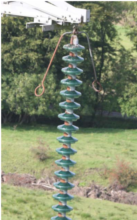
Figure 13: level of rust at ZP Route insulator sets
