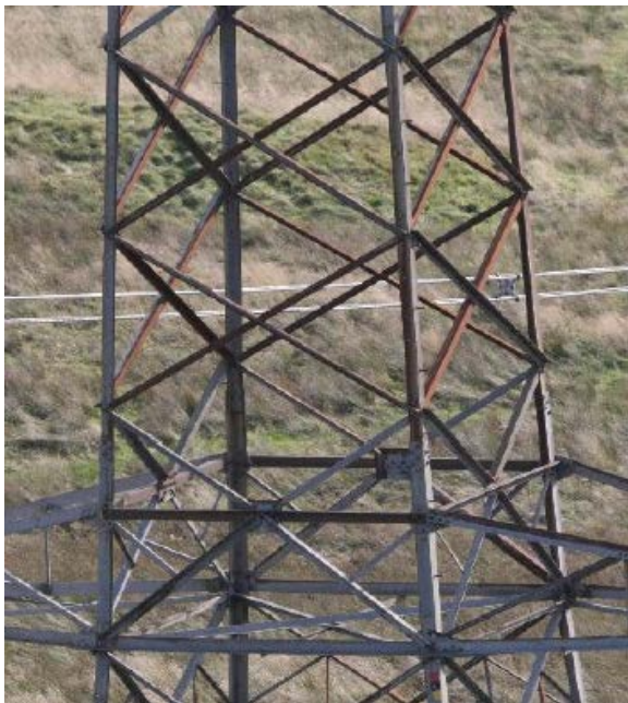
Figure 16: severely rusted ZP017.
