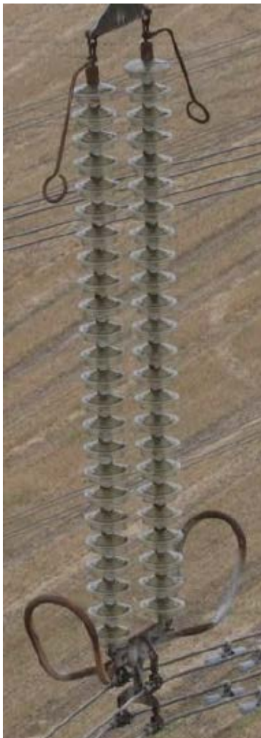
Figure 4: rust degraded suspension insulator set at ZC(S) Route.
