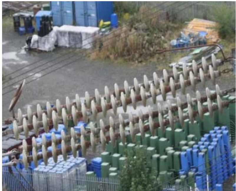
Figure 26: tension insulator severely rusted and degraded mechanical caps at ZC(N) Route.
