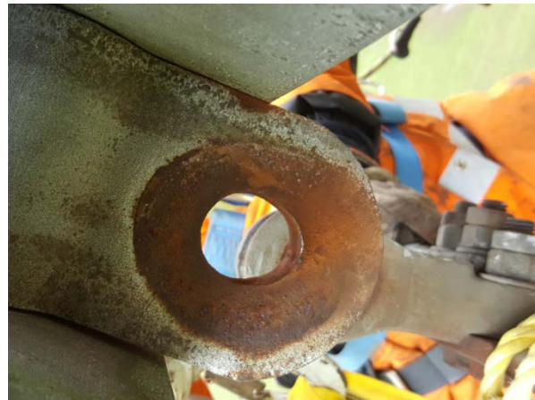
Figure 12: worn suspension connection at ZP008
