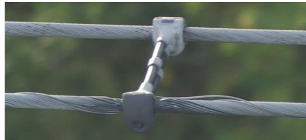
Figure 20: conductor damage at spacer clamping position at ZF 141-142.
