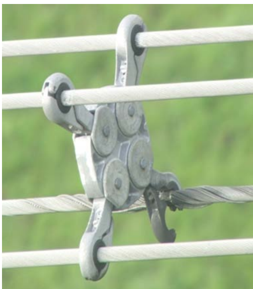
Figure 9: conductor damaged at 'Dunlop' spacer-damper clamping position at ZP Route (074-075).
