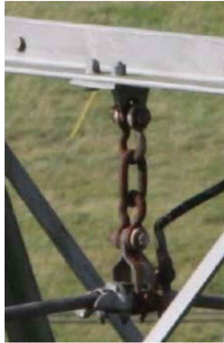
Figure 15: worn of earth wire suspension connection at ZP005
