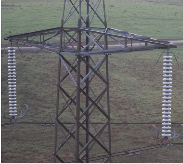
Figure 30: level of rust through towers along ZS Route.
