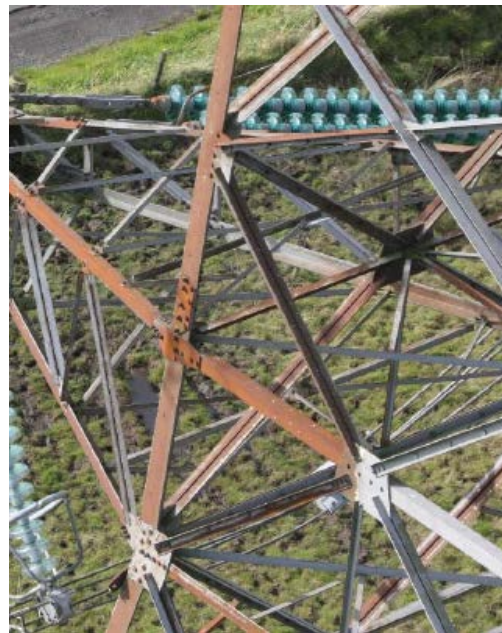
Figure 17: severely rusted cross-arm ZP007.
