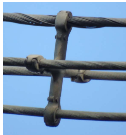
Figure 10: conductor damaged at jumper spacer clamping position at ZP Route (068).
