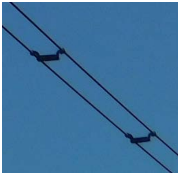
Figure 28: slipped spacer.
