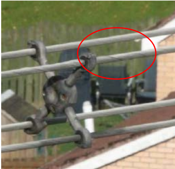
Figure 1: conductor damaged at ‘Andre’ spacer clamping position at ZD Route.
