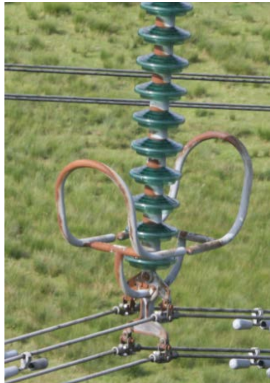
Figure 12: worn suspension connection at ZP008
