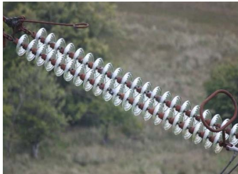
Figure 22: tension set at ZF Route.
