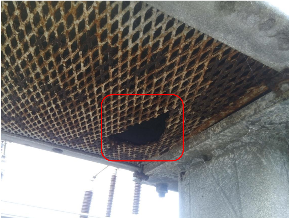
Figure 3-7 - Example of corrosion of disconnector at St Fergus Mobil – note holes in the steel cross member
