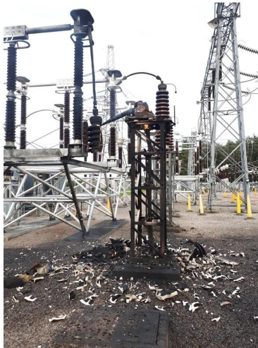
Figure 9 - Kintore 275kV Cable Sealing End Failure
