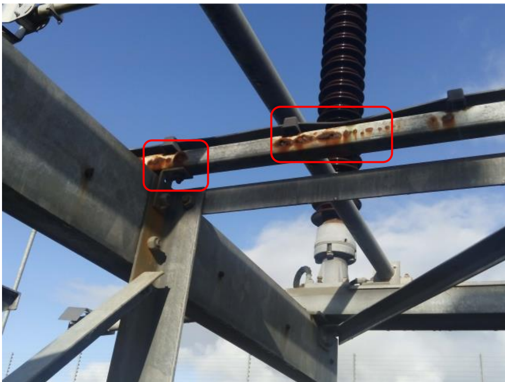
Figure 3-7 - Example of corrosion of disconnector at St Fergus Mobil – note holes in the steel cross member
