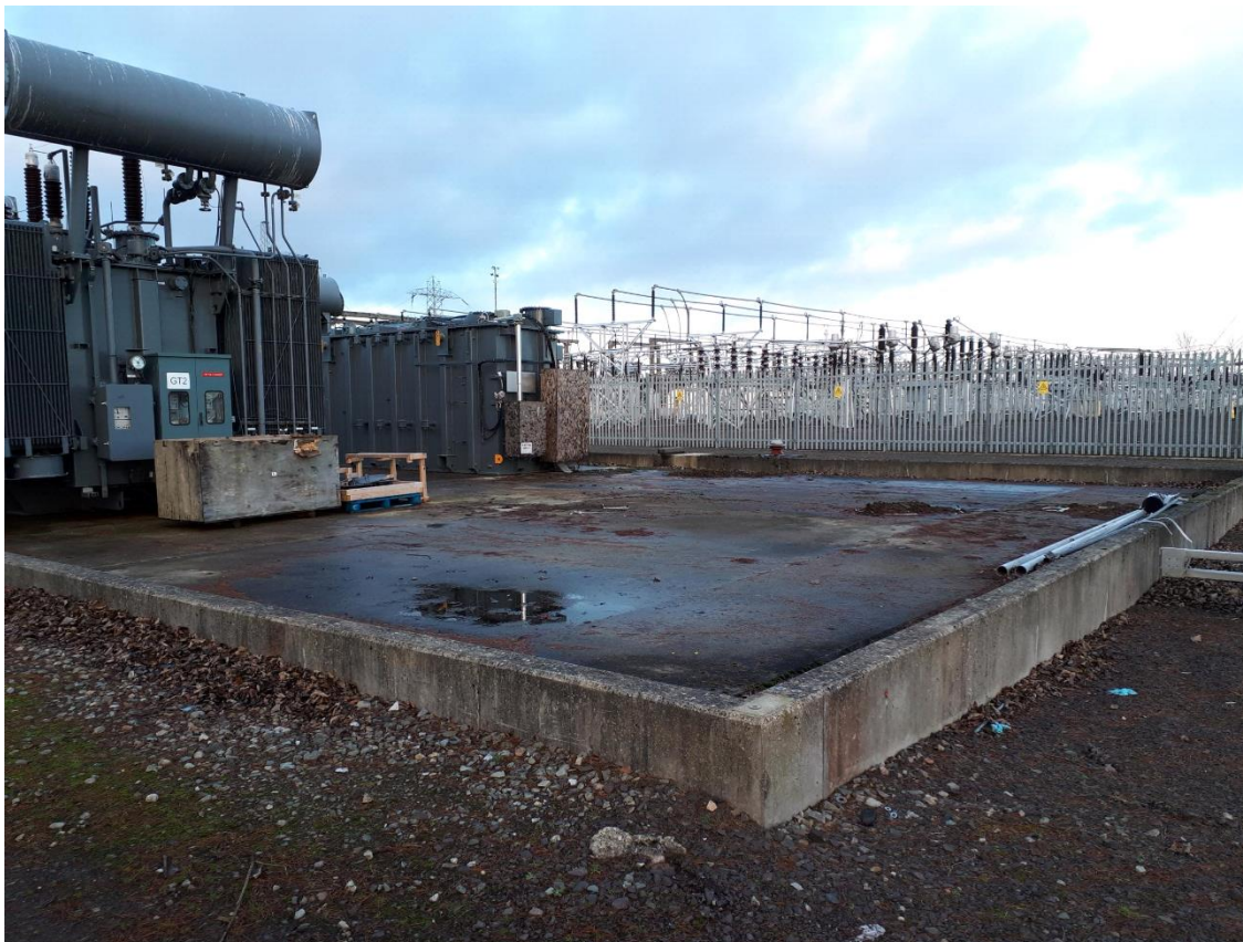
Figure 21 - Poor bund condition in an exposed location in proximity to a live HV zone
