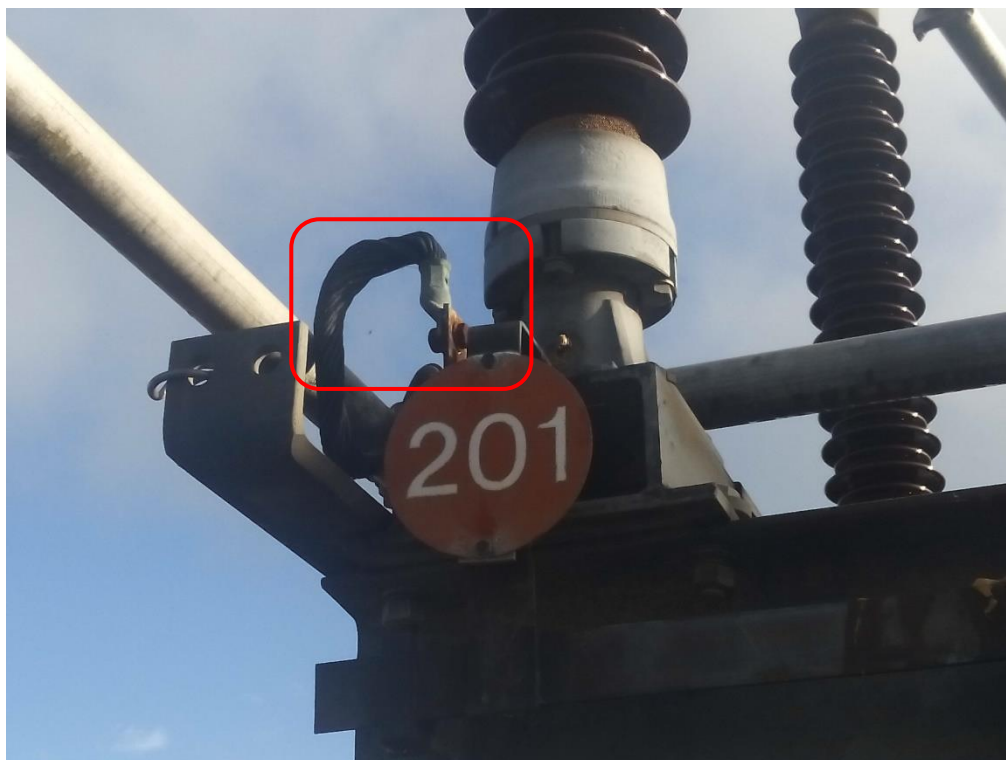
Figure 3-9 - Example of corrosion of disconnector at St Fergus Mobil – note the corrosion on the safety critical earth braid
