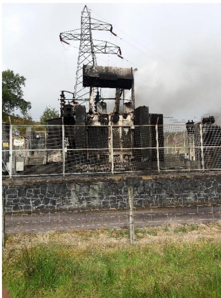
Figure 3 - Nant Transformer Failure – GT1 2017
