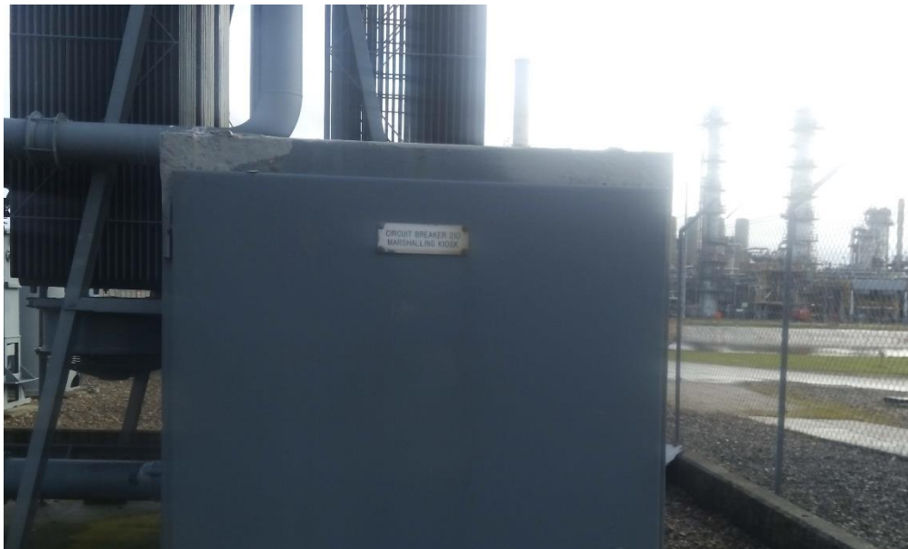
Figure 3-11 - Example of corrosion of marshalling kiosk at St Fergus Mobil – note top of kiosk and gas plant in background
