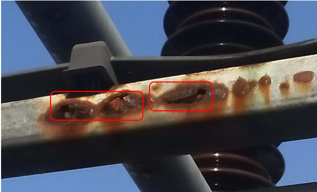
Figure 3-9 - Example of corrosion of disconnector at St Fergus Mobil – note the corrosion on the safety critical earth braid
