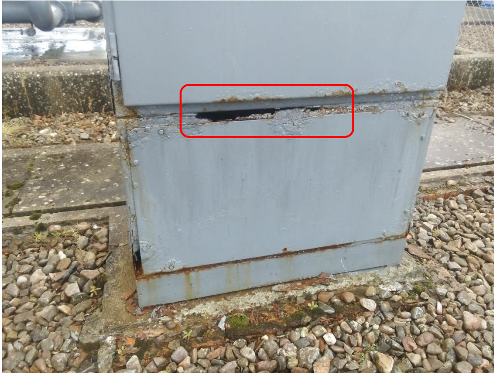
Figure 3-11 - Example of corrosion of marshalling kiosk at St Fergus Mobil – note top of kiosk and gas plant in background
