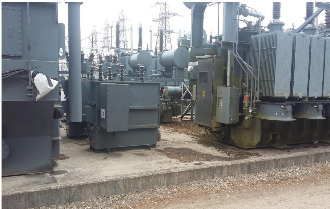
Figure 24 - Stored Grid transformers are degrading due to weather conditions
