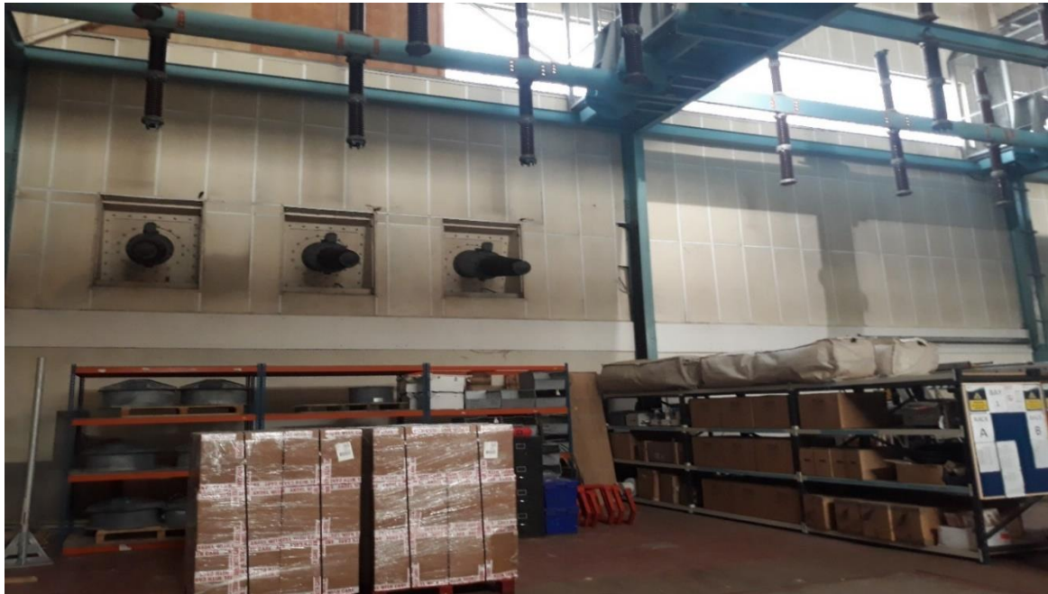
Figure 15 - Wall bushings that require removal
