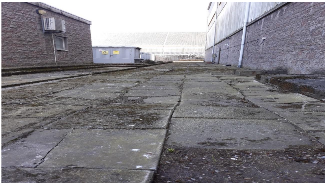
Figure 19 - Exterior side of building is limited as this was previously a cable trench for major cables and will need significant investment to be load bearing.
