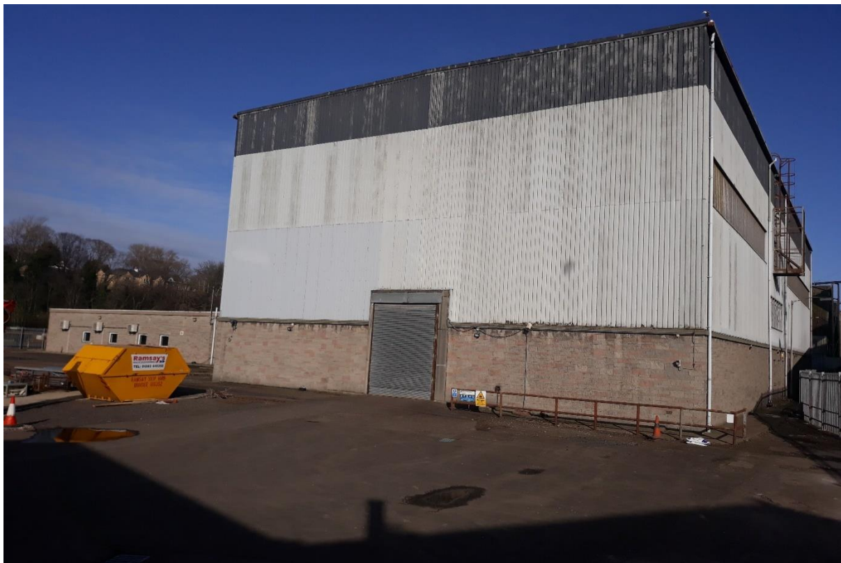
Figure 16 - The access to the building is limited due to the current door dimensions. This is the only vehicular access.
