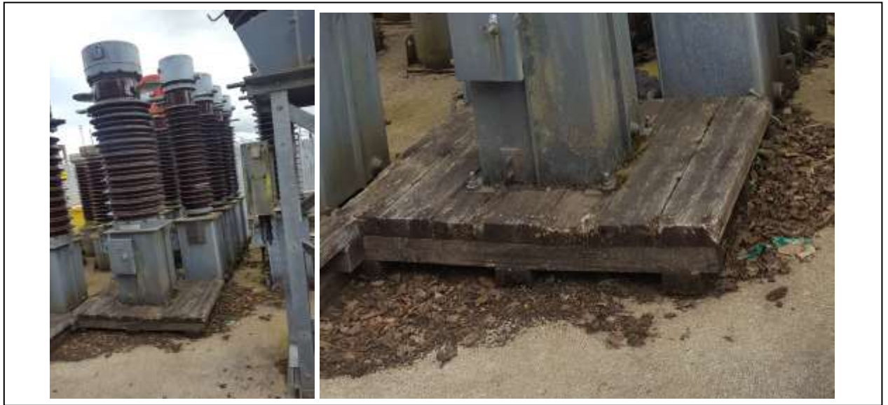
Figure 20: Tealing - Pallet Deterioration
