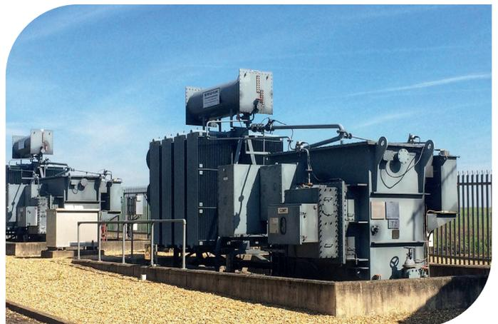
Figure 19: Two 33/11kV primary substation transformers during a visit to a LEAN project trial site
