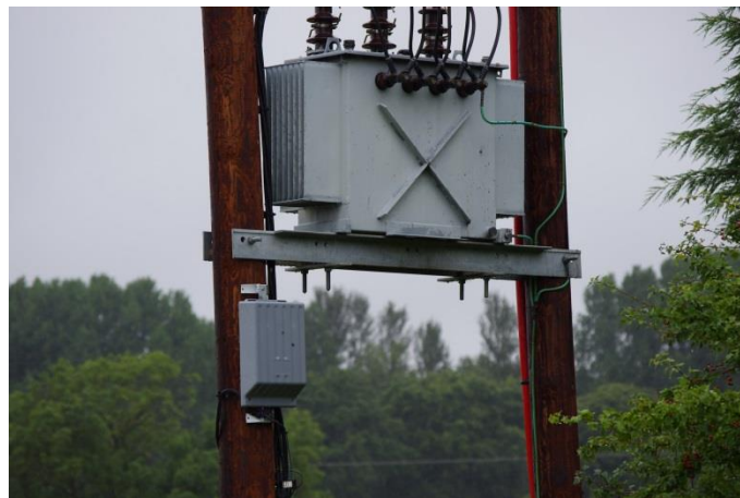
Figure 26. ESSM device installed in SPEN outdoor substation
