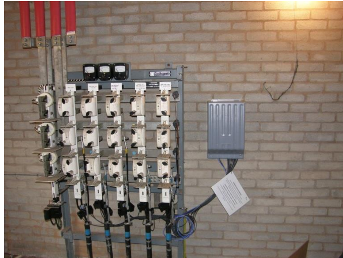
Figure 25. ESSM device installed in SPEN indoor substation
