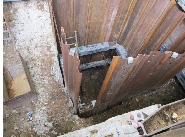
Figure 2: A 5½ meter deep £78k trial hole
