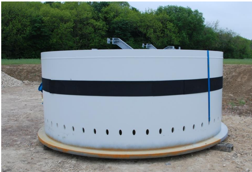
Figure 2-4 Wind Turbine Transition Piece (waiting to be installed), Showing Black Neoprene Strip
