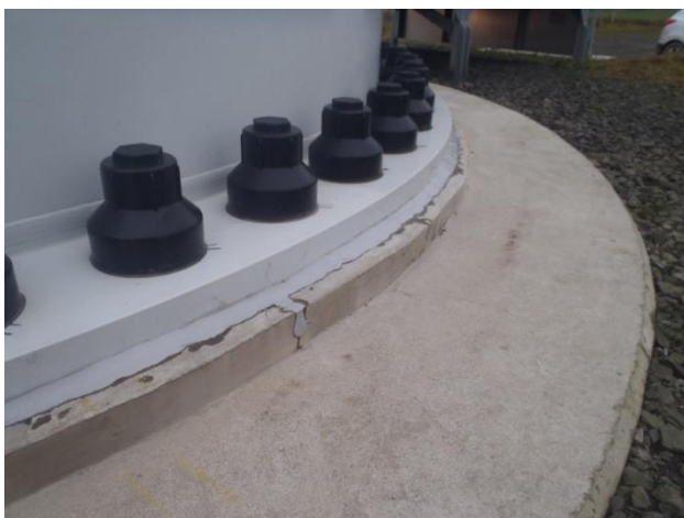
Figure 2-3 Example of Rubber Caps on External Bolted Connection
