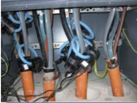
Figure 5 Flexible Rogowski coils 'live installed' at two LV feeders
