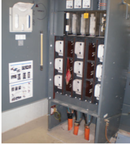
Figure 5 Flexible Rogowski coils 'live installed' at two LV feeders
