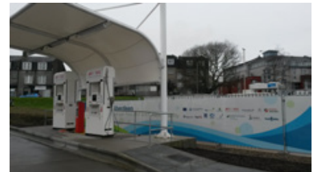
Figure 15 Kittybrewster Hydrogen Refuelling Station, Aberdeen
