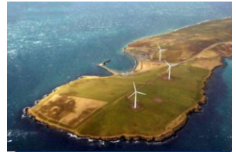
Figure 11 Spurness windfarm Orkney
