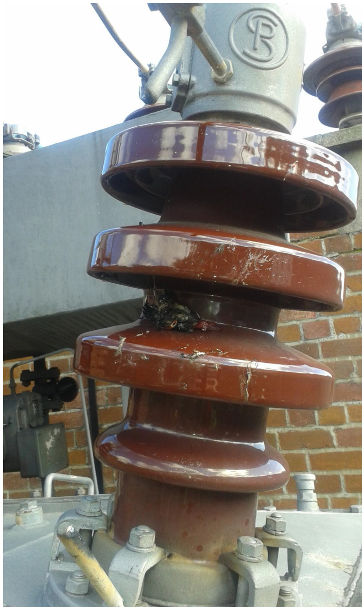
Photograph 4 – a close-up of the 33kV bushing and exposed arcing horns
