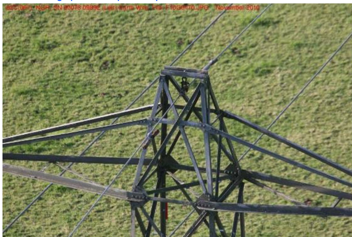
Photograph 6 – the apex clamp at tower C67 as seen in November 2010
