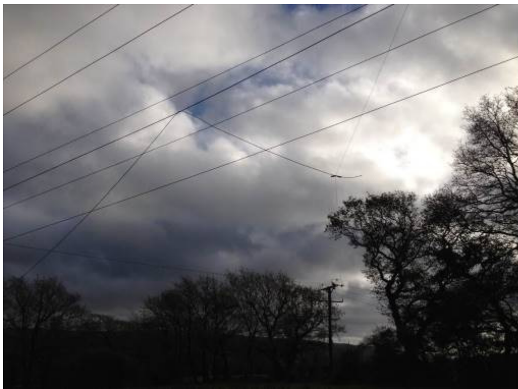
Photograph 5 - the failed earth wire lying on the number one 132kV circuit and on the under-running 11kV overhead line
