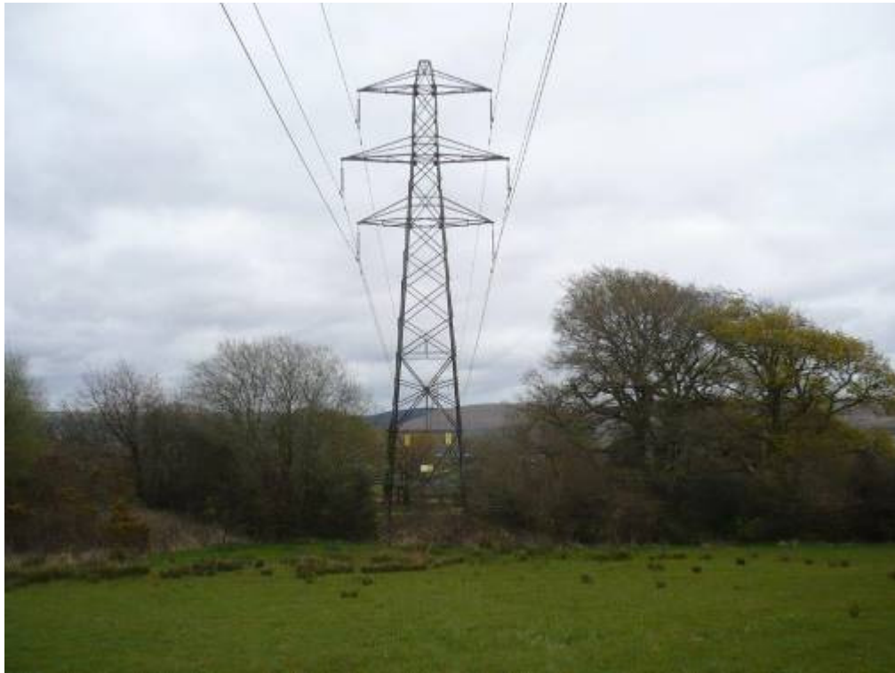
Photograph 7 - a view of tower C67 showing the disposition of the cross arms
