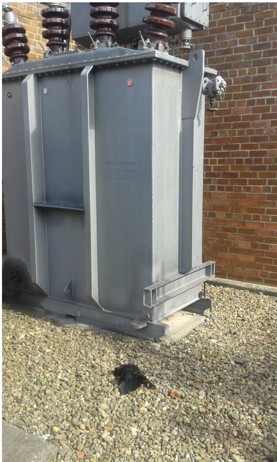
Photograph 3 – the dead crow in relation to the number two 33kV auxiliary earthing transformer
