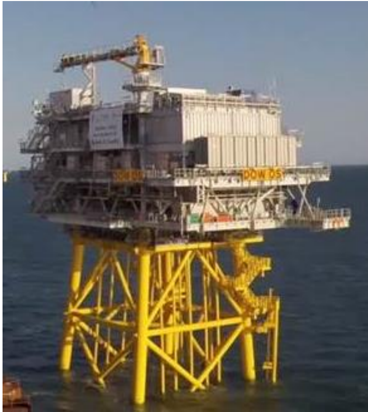
Dudgeon Offshore Substation; successfully installed on 07 August 2016
