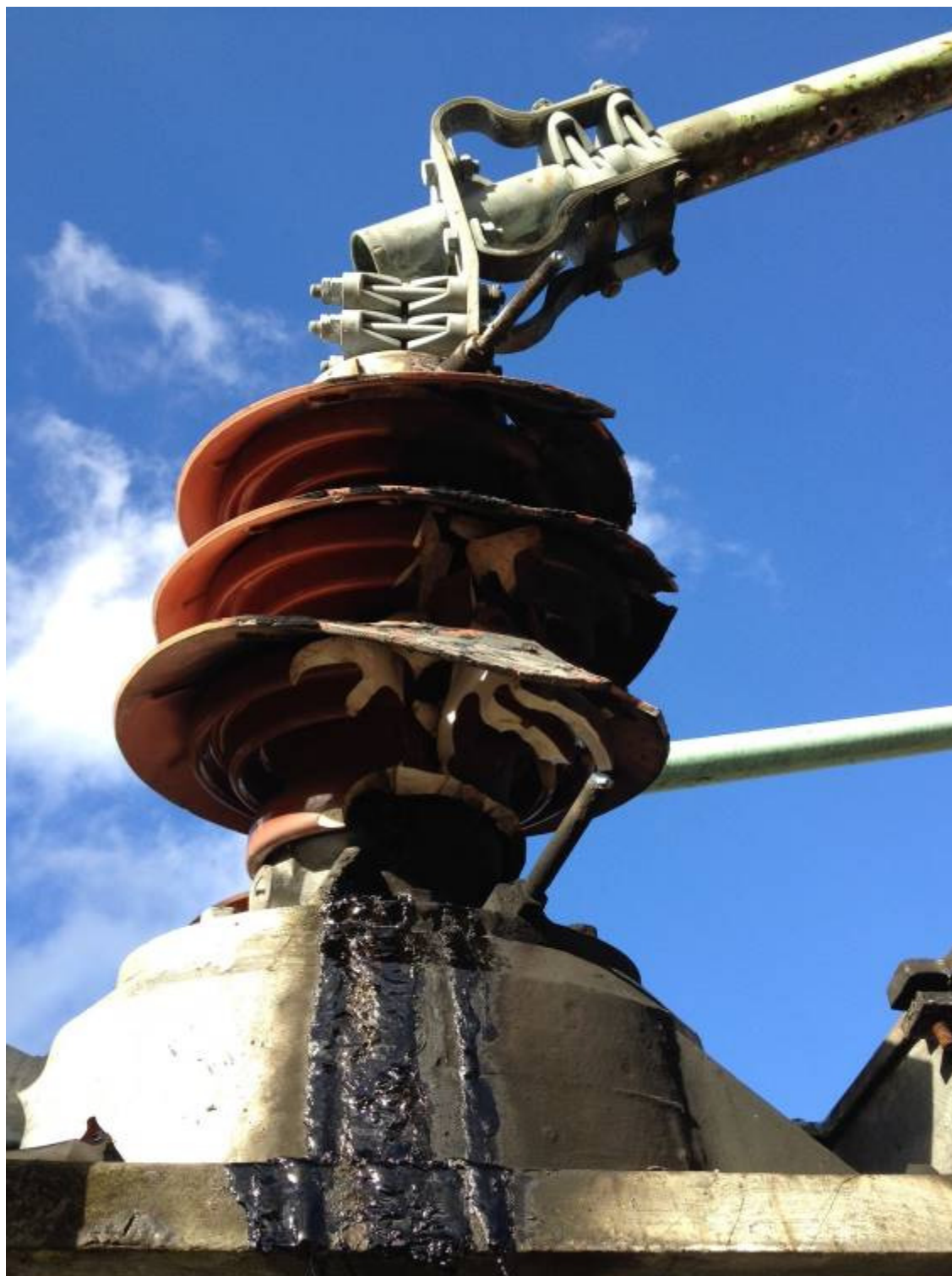
Photograph 2 – Close-up of the irreparably damaged bushing
