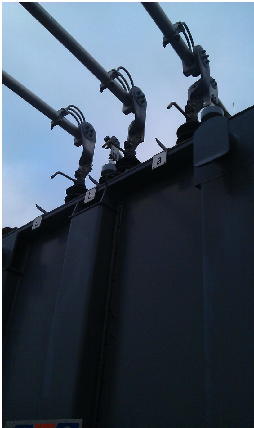
Photograph 3 – The exposed 33kV connections of the number 1 132/33kV Grid Transformer at the time of the incident
