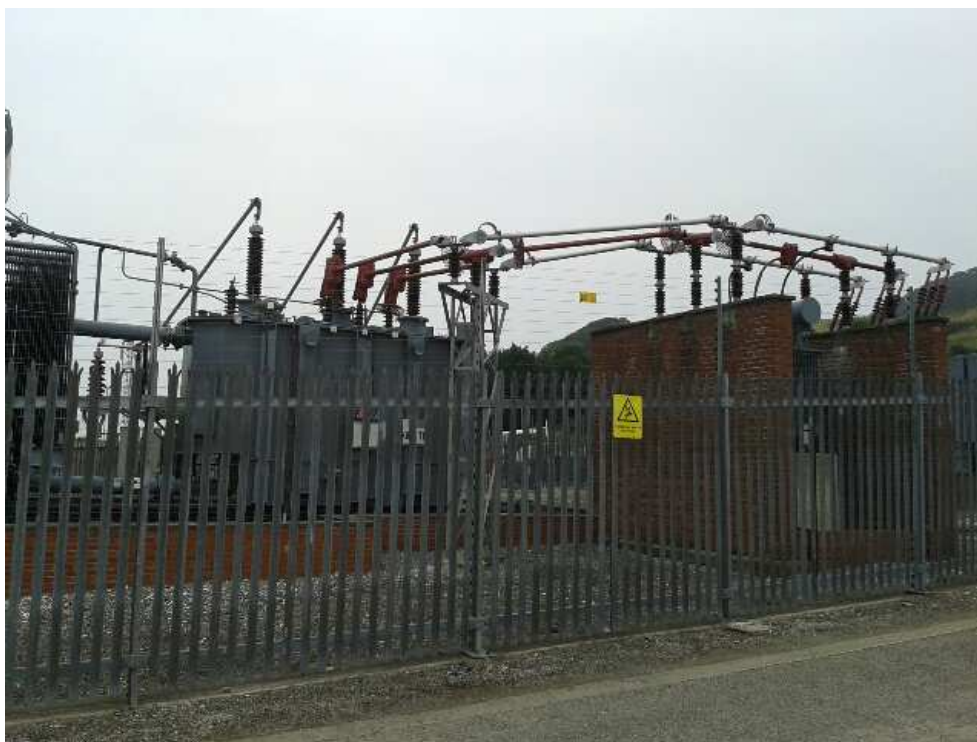
Photograph 5 - A close-up of the fence surrounding NPG's 132/33kV Scarborough Grid Substation showing the electrified wire extension above the 2.4 metre-high 'unclimbable' palisade palings
