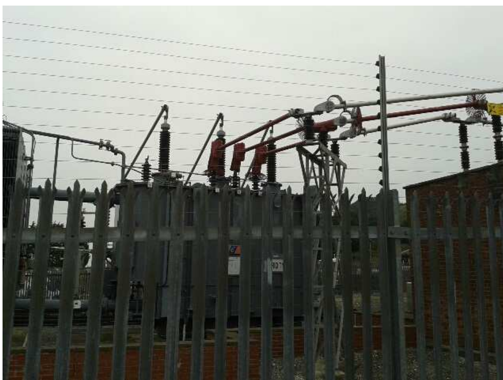
Photograph 5 - A close-up of the fence surrounding NPG's 132/33kV Scarborough Grid Substation showing the electrified wire extension above the 2.4 metre-high 'unclimbable' palisade palings
