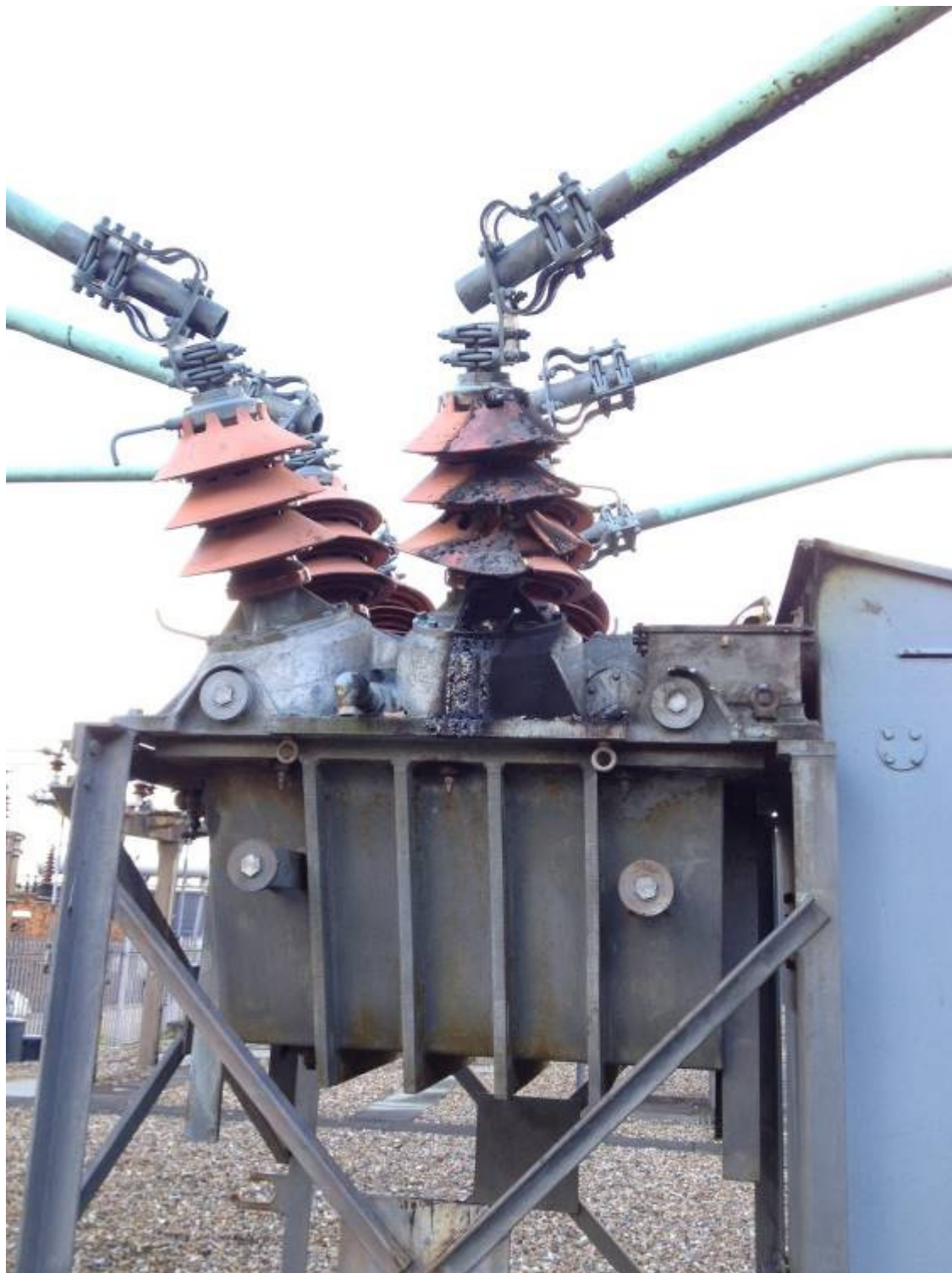
Photograph 1 – The irreparably damaged bushing and its associated 33kV circuit-breaker
