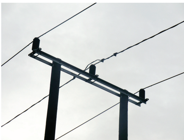
Figure 13 – Fibre wrapped OHL (middle conductor)
