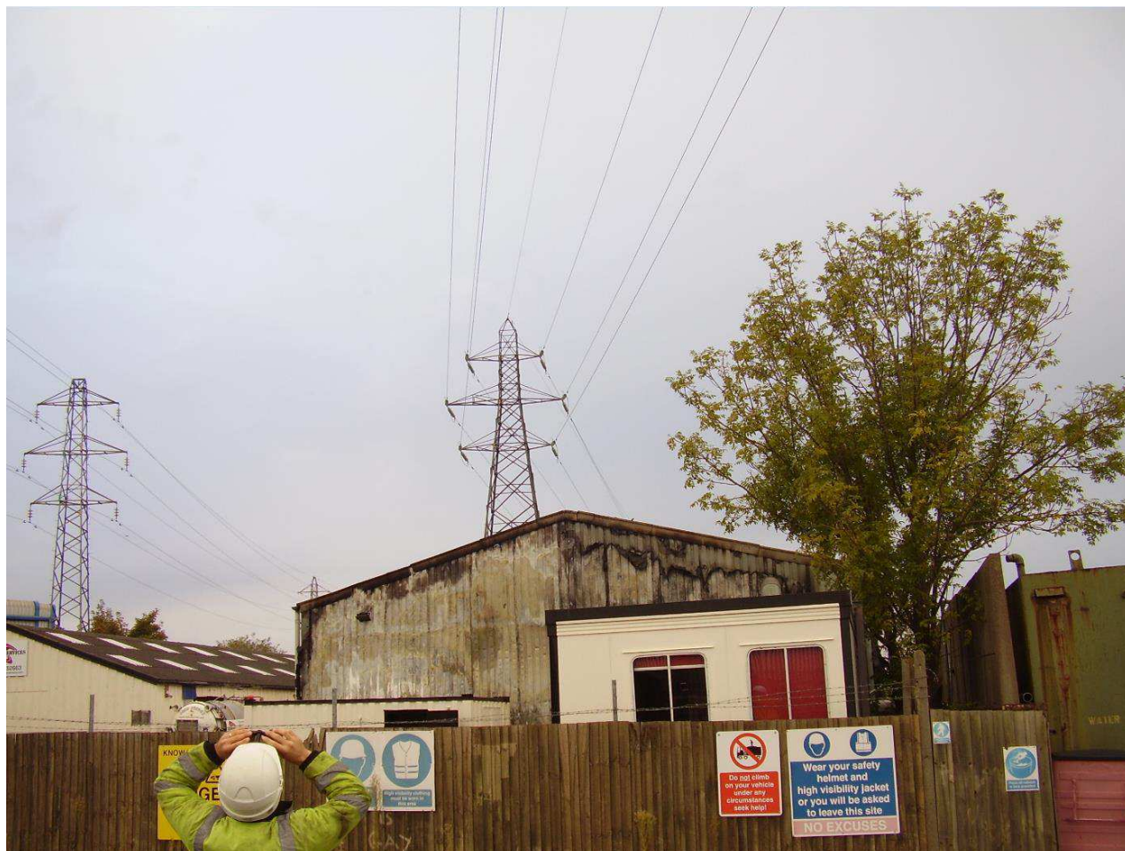
Photograph 1 – 'End-on' view of the 132kV double-circuit overhead tower line and the fire-damaged building below
