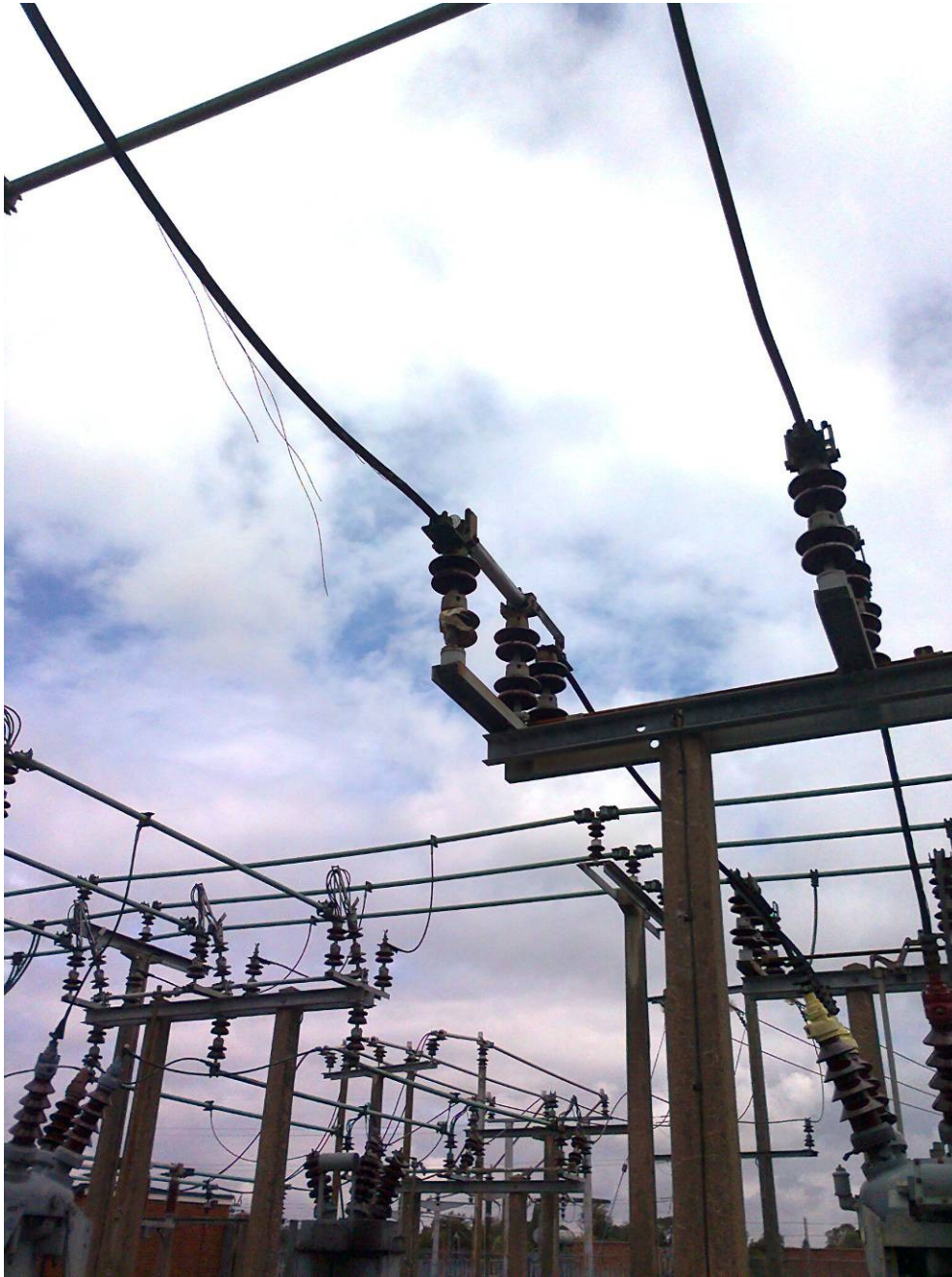
Photograph 1 – View of 33kV isolator C1W6 showing the remnants of the metallised tail of the balloon dangling from the overhead connection and the in-situ irreparably damaged post-type insulator
