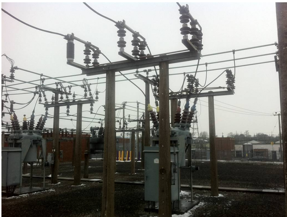
Photograph 3 – View of 33kV isolator C1W6 following replacement of the irreparably damaged post-type insulator
