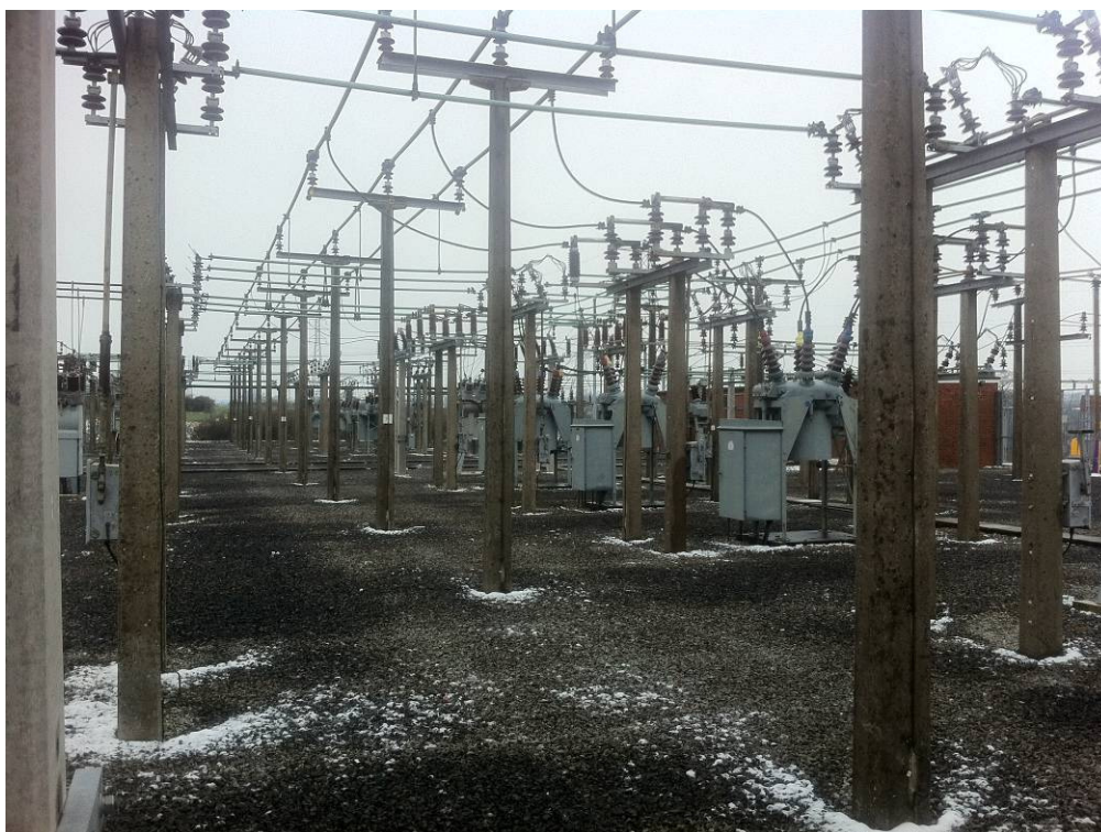
Photograph 3 – View of 33kV isolator C1W6 following replacement of the irreparably damaged post-type insulator
