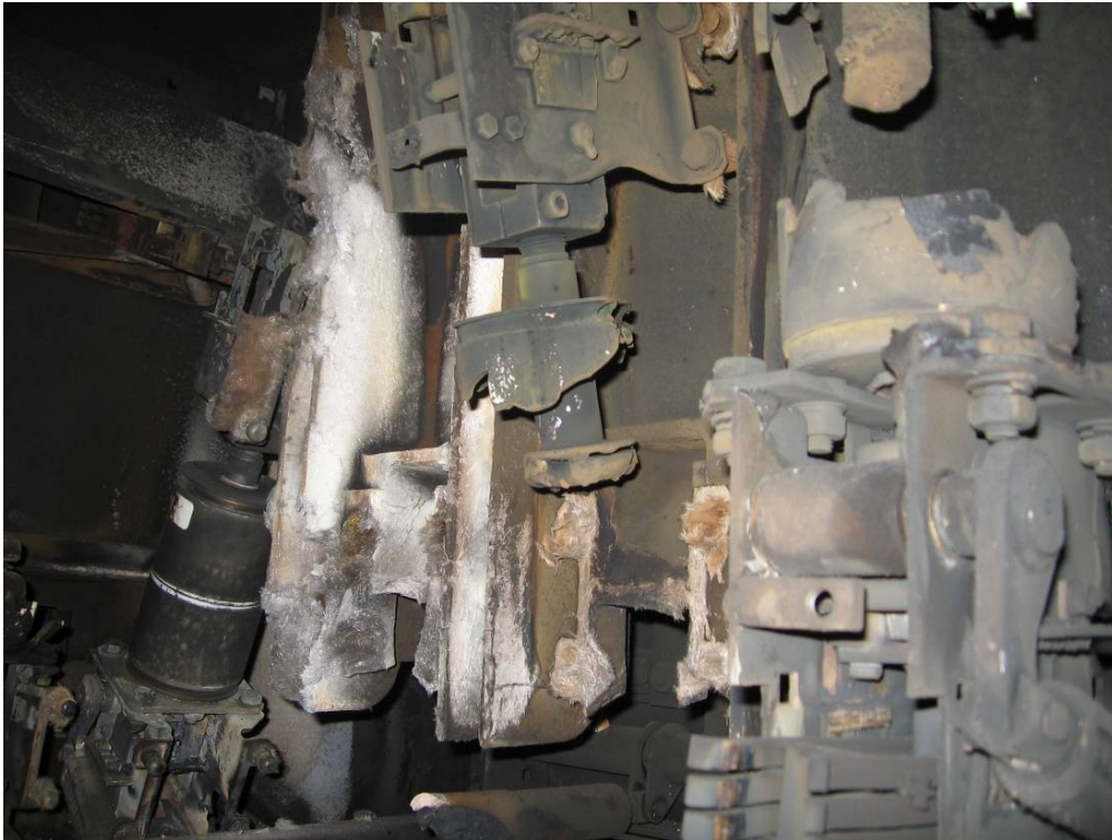
Photograph 1 – The damaged 11kV vacuum circuit-breaker
