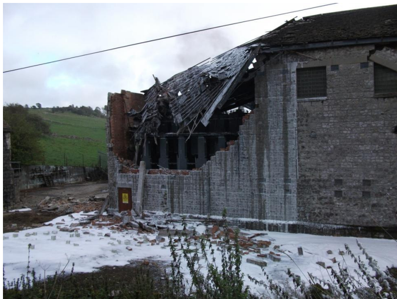
Photograph 1 – The damage to the 33kV switchhouse
