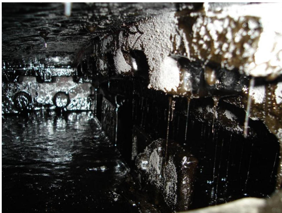
Photograph 2 – The faulted busbar chamber
