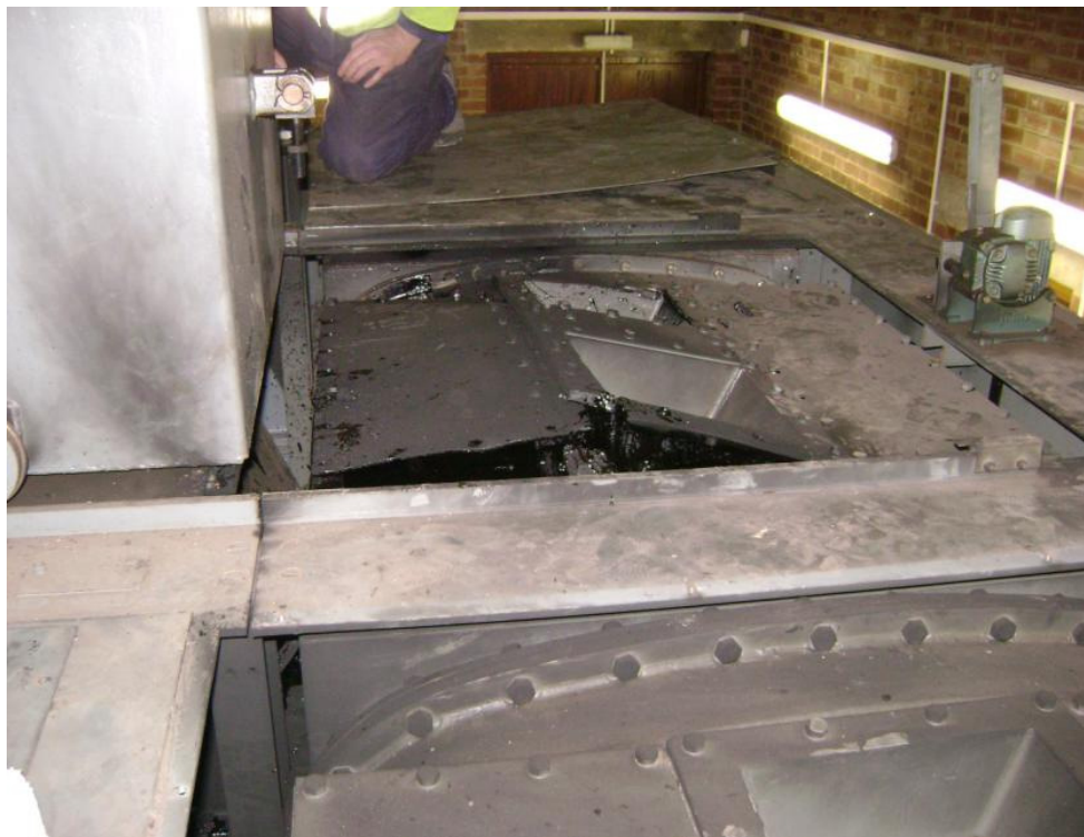
Photograph 1 – The cover plates above the faulted busbar
