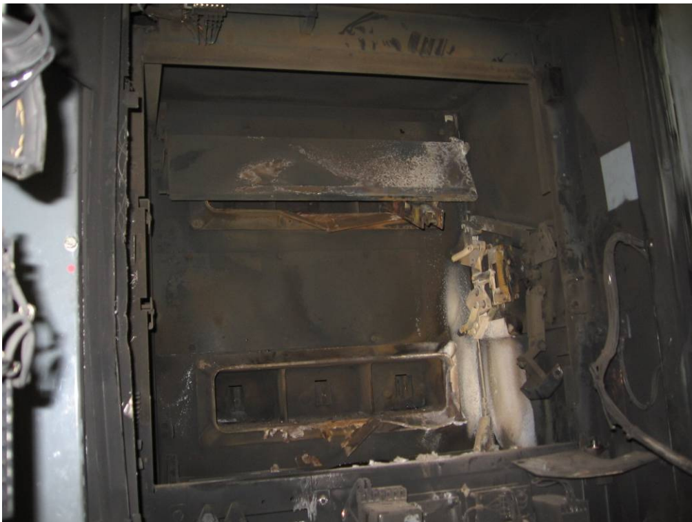
Photograph 2 – The damage to the fixed portion of the Parliament Street 11kV circuit-breaker housing
