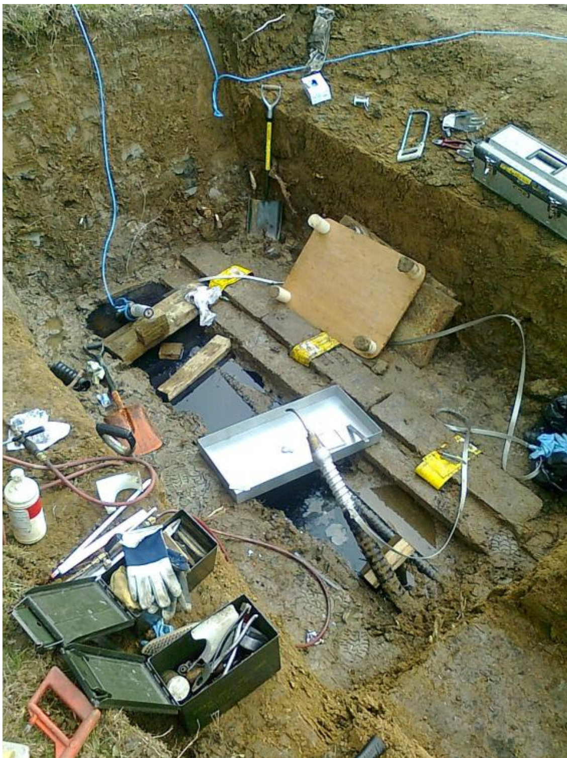
Photograph 3 – The repair work in progress – the concrete cable files protecting the cables are clearly visible
