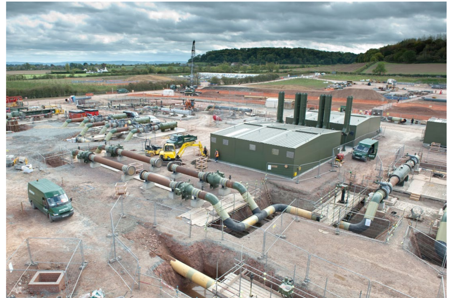
Pipework under construction at a High Pressure installation.
