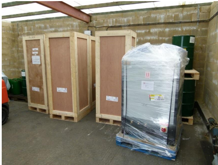
Figure 3. Showing first Multi Terminal PED delivered to an SPN Substation
