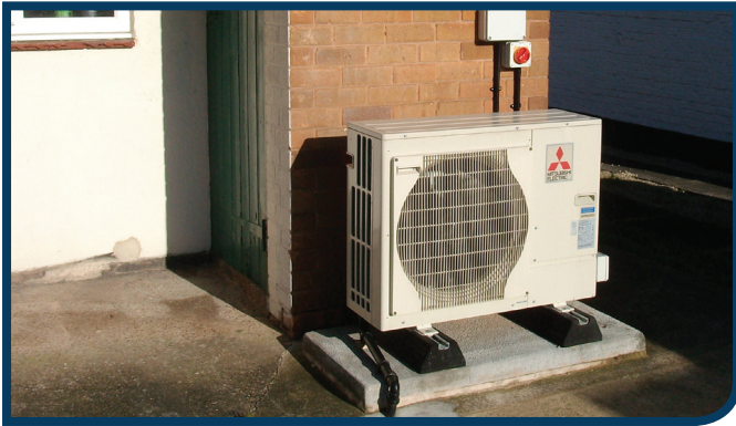
ASHP project in Yarwell.
