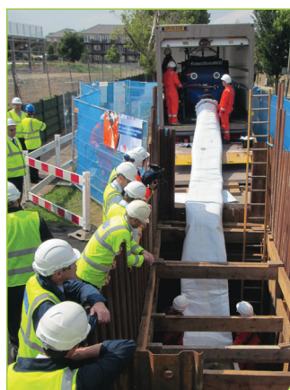
The CIPP technique being monitored by engineers.
