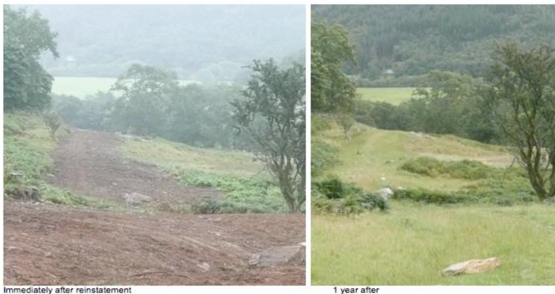
Hafod y Llan, Snowdonia hydro site a year after installation – a 660mm diameter pipe buried here
