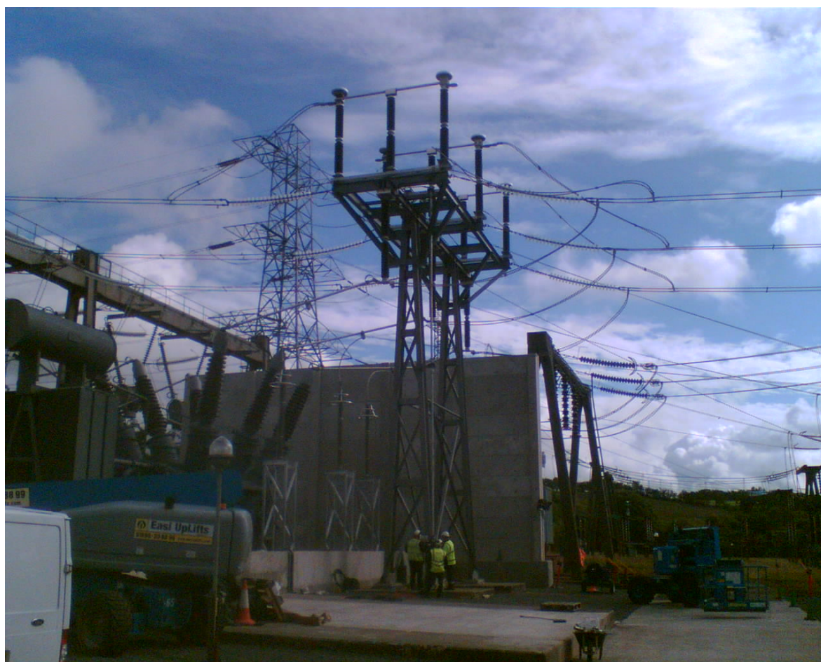
Figure 4.11 – 275kV Series Reactor on Neilston Circuit (Under Construction)
