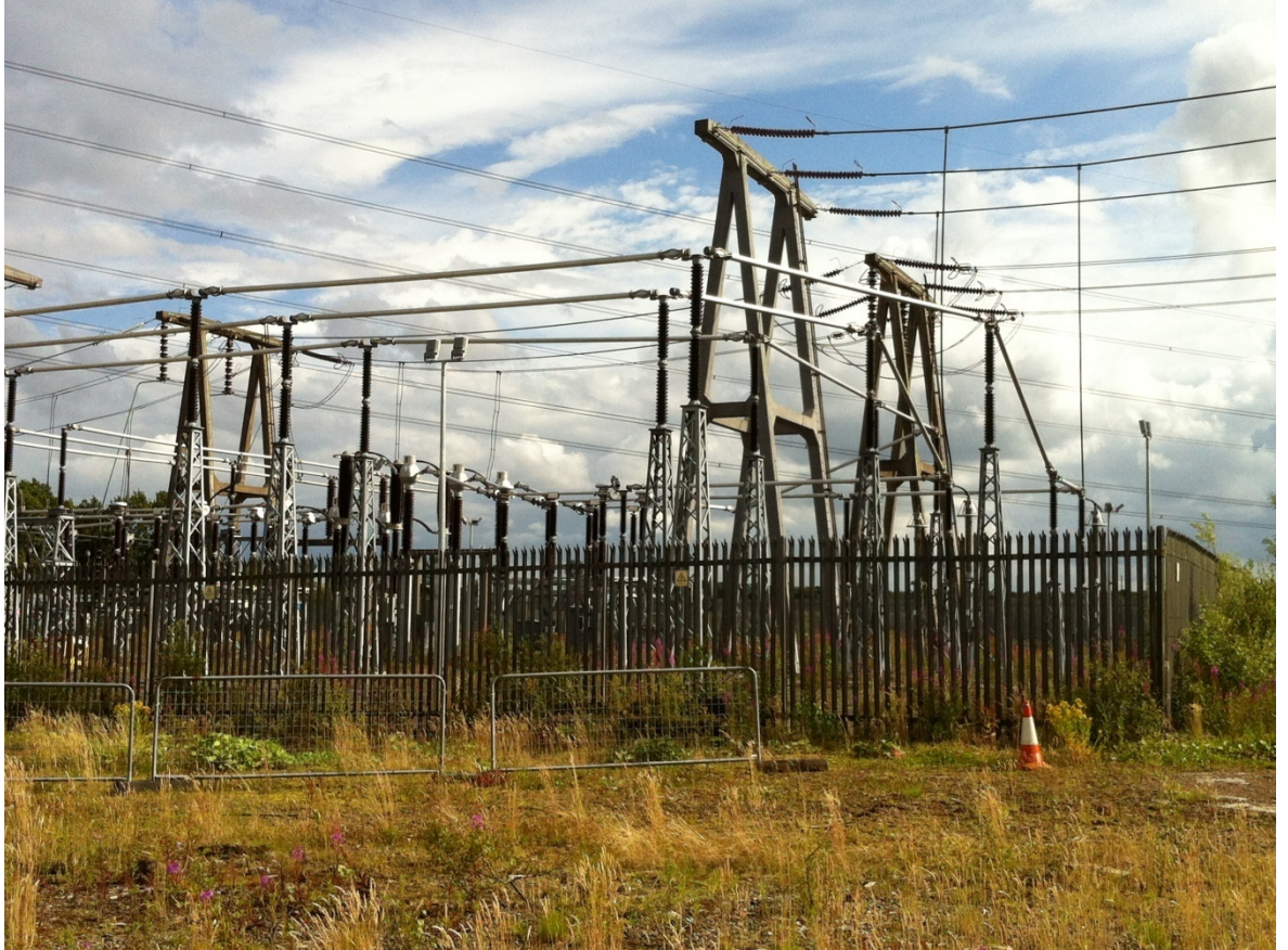
Figure 4.7 – Mesh Corner 1 and Single Switch Circuit Breaker
