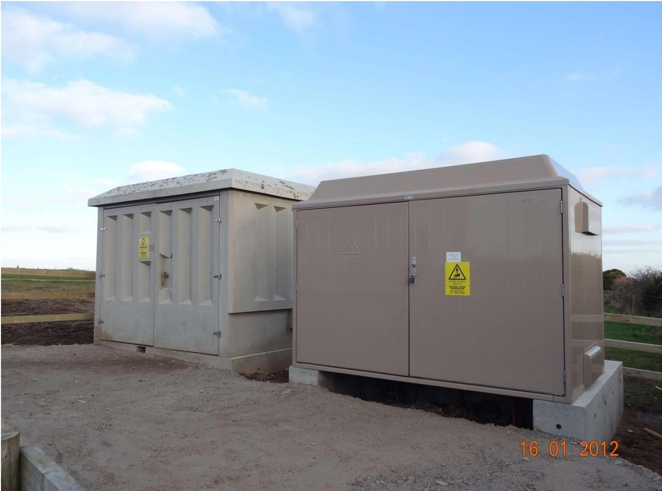
Figure 8: D-SVC (left) and associated transformer (right) installed on site
