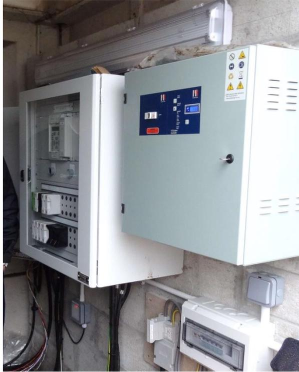
Figure 4: Voltage protection relay, battery and battery charger in situ
