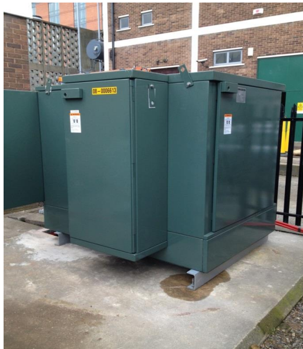
Figure 5-8: Pad-Mounted Style IntelliRupter® PulseCloser on site
