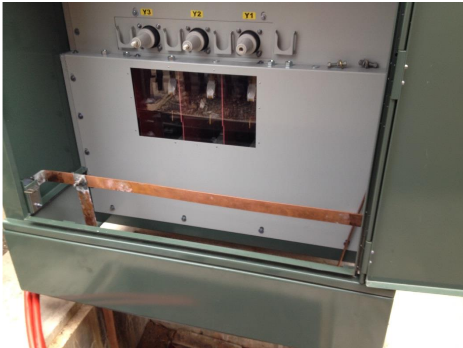
Figure 5-12: Earth bar upgrade of Pad-Mounted Style IntelliRupter® PulseCloser
