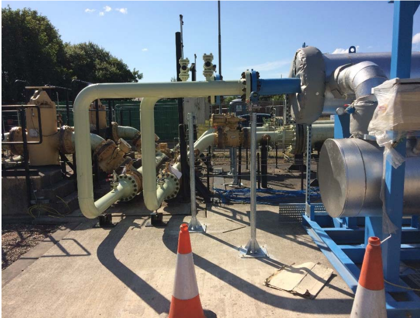
Figure 5. Small LP Steam unit installation at Low Moor
