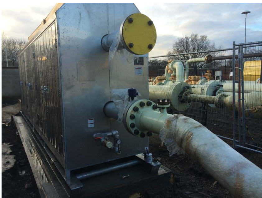
Figure 2. Installation of the small Hotcat at Crossgates
