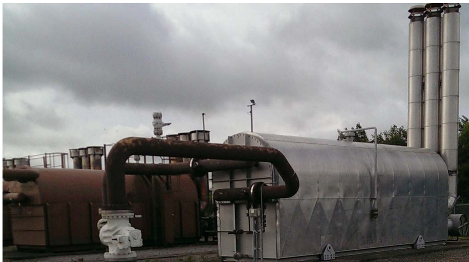
Figure 8. WBH's at Pannal where additional instrumentation has been installed
