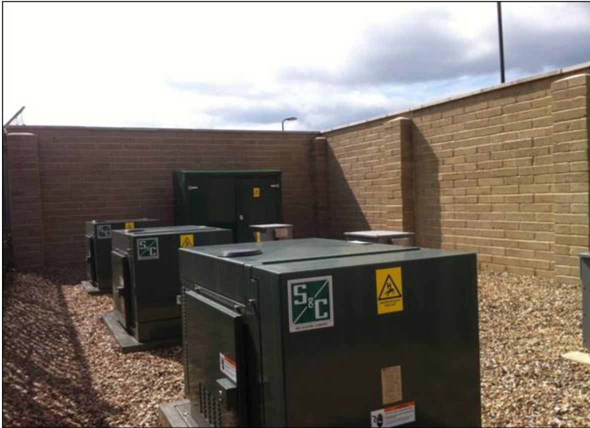
Figure 15 - Internal view of completed site
