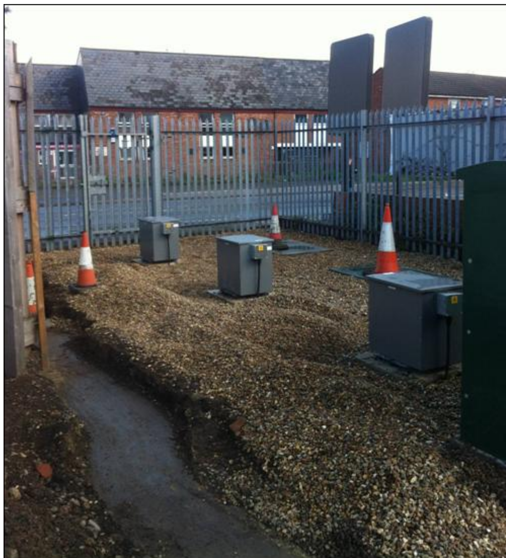
Figure 13 - Site levelled with transformers and distribution cabinet installed
