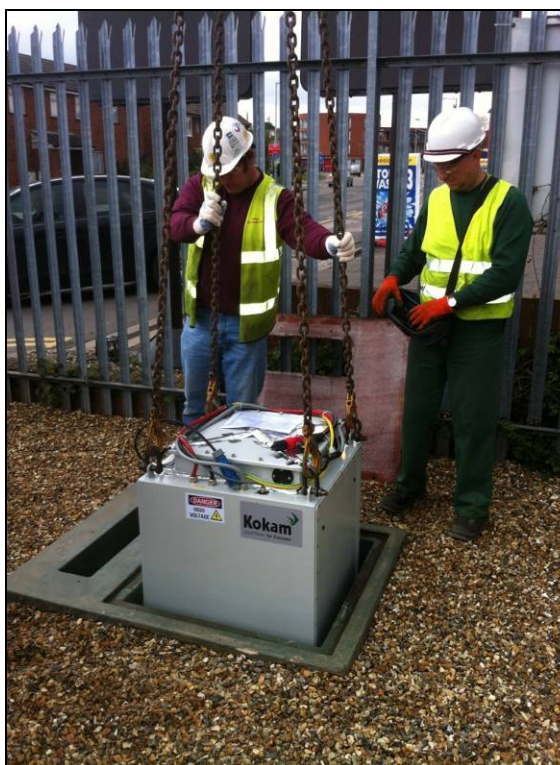
Figure 2: Battery being lowered into vault on site
