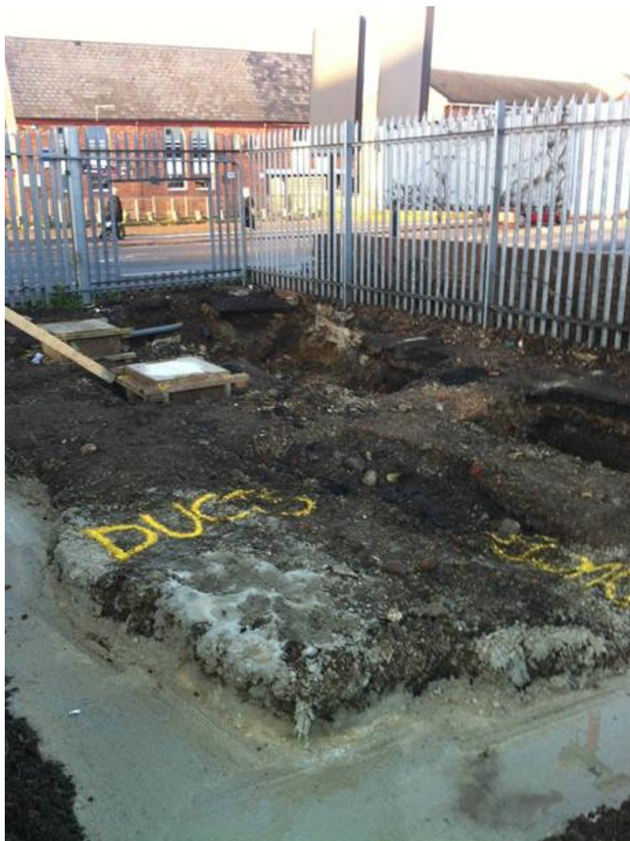
Figure 11 - Site after initial excavations and perimeter wall foundations
