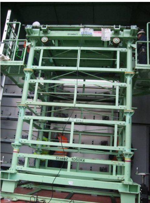
Figure 16 - Battery insertion tool at full height
