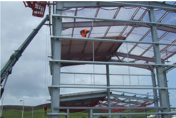
April – External building frame erected
