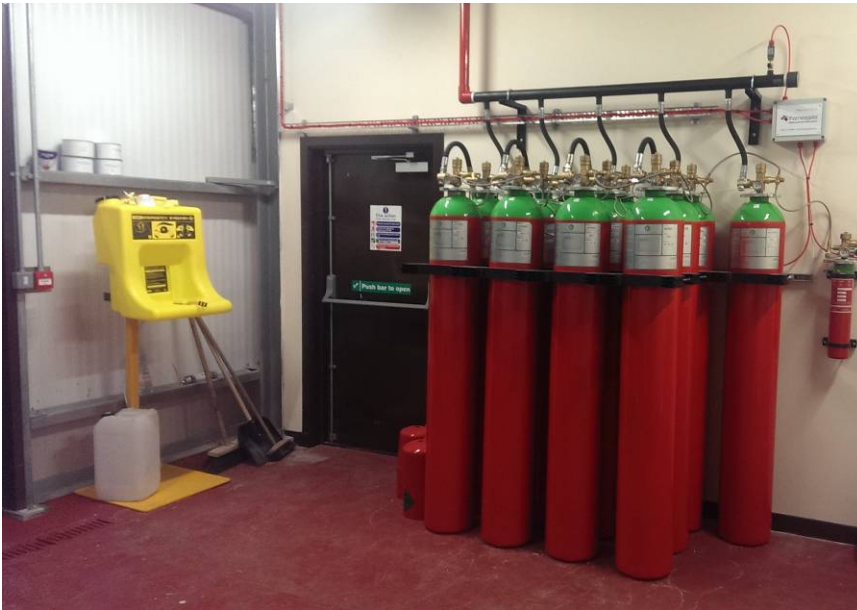
Figure 31 - Inert gas for fire suppression
