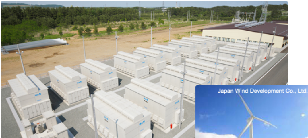
Figure 1 - 34MW NAS battery
