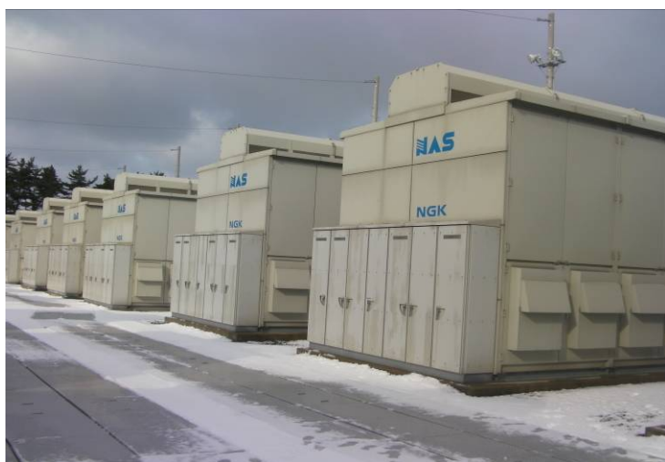
Figure 5 - 34MW battery, Rokkasho wind farm, Japan
