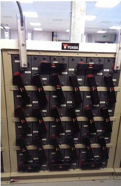
Figure 24 - VRLA battery rack
