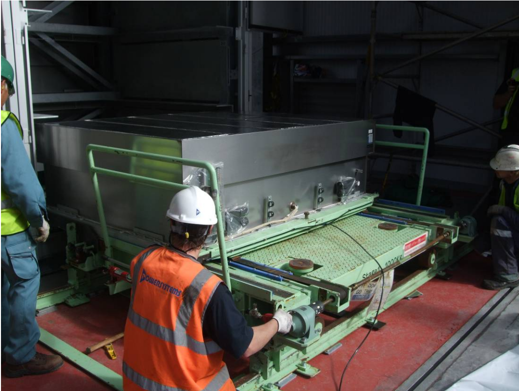
Figure 13 - Battery module insertion
