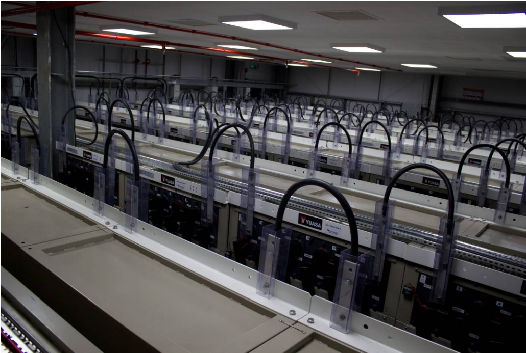
Figure 27 - Installed battery (i)
