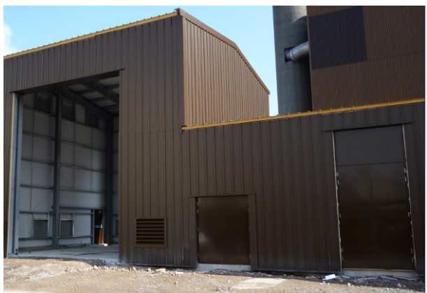
May – Building fully clad, internal works begin
