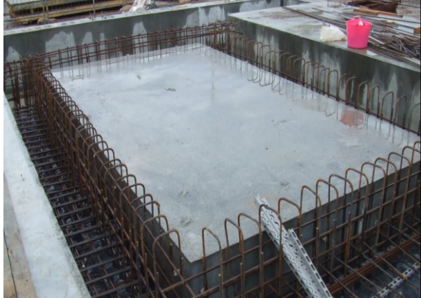
March – Concrete and rebar laid, foundations complete
