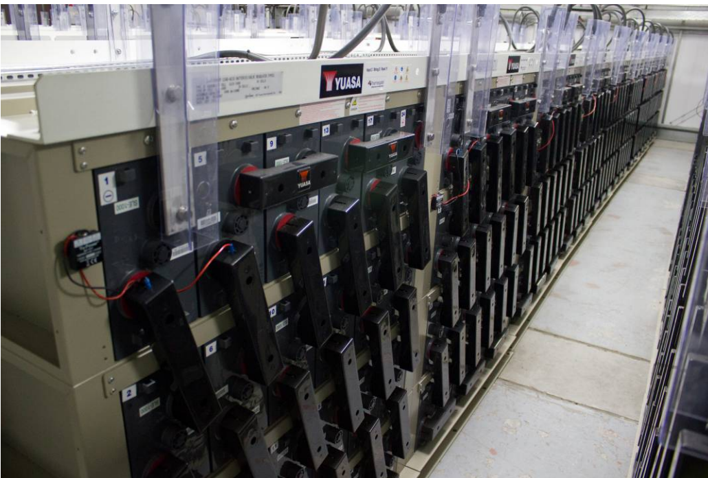
Figure 28 - Installed battery (ii)
