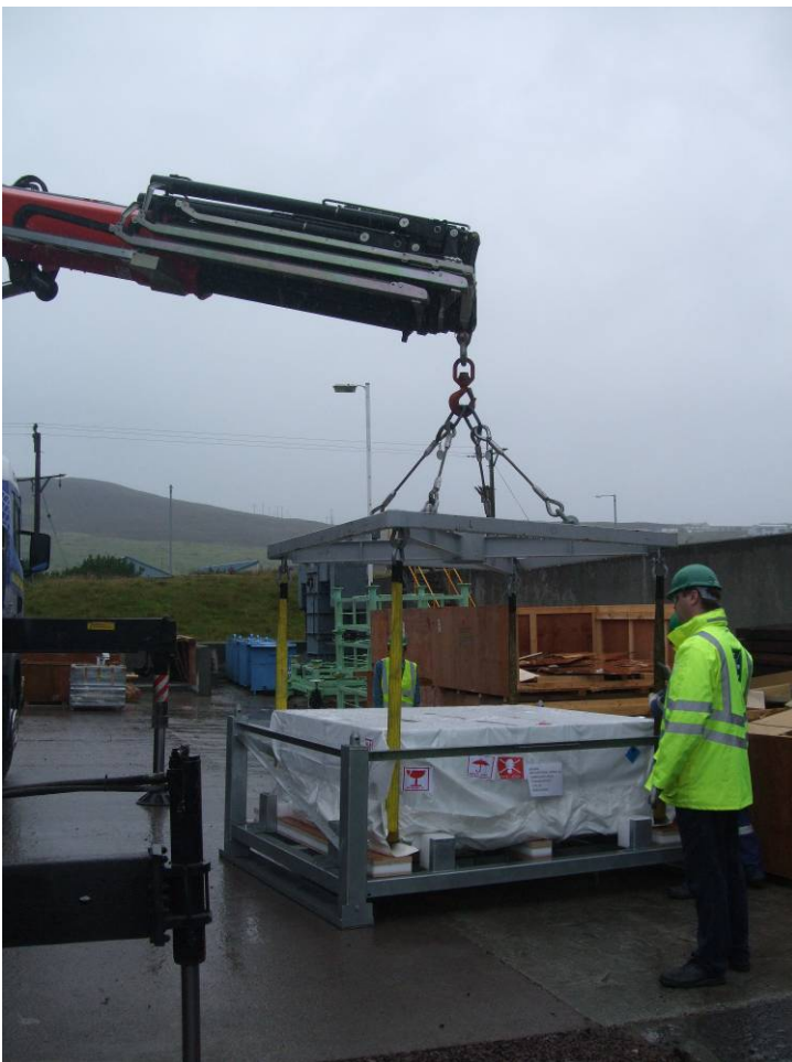
Figure 12 - Battery module being removed from transportation frame
