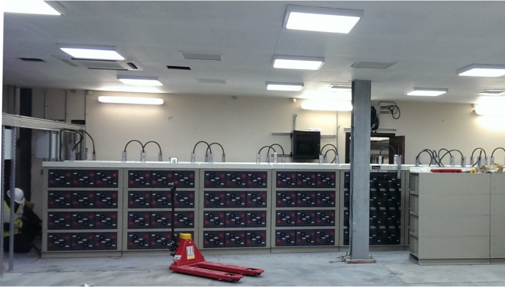
Figure 23 - VRLA battery installation
