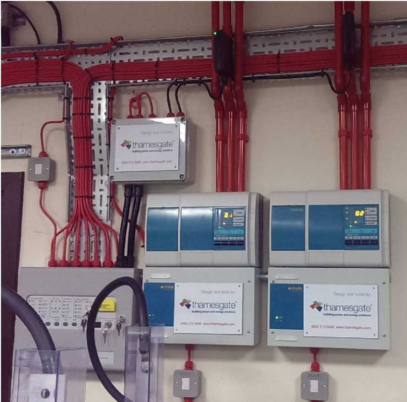
Figure 30 - VESDA and hydrogen detection
