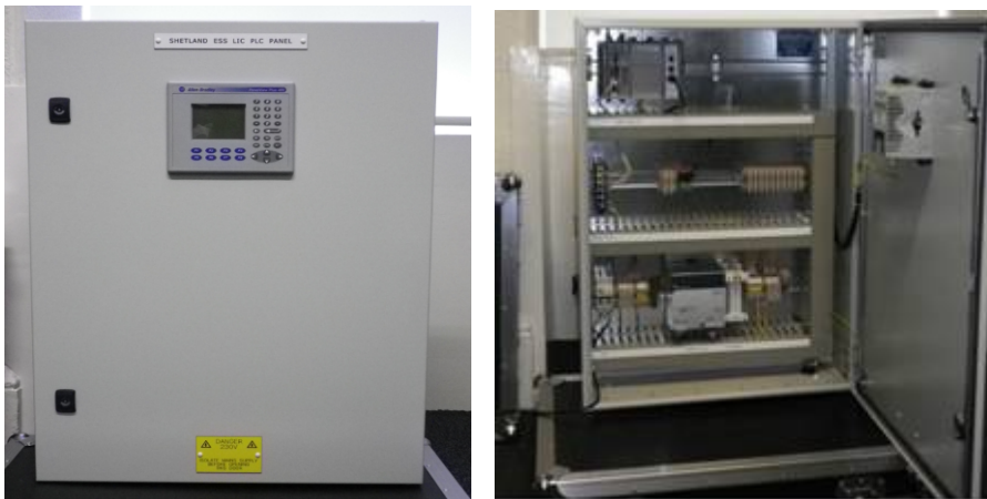
Figure 19 - Local interface controller
