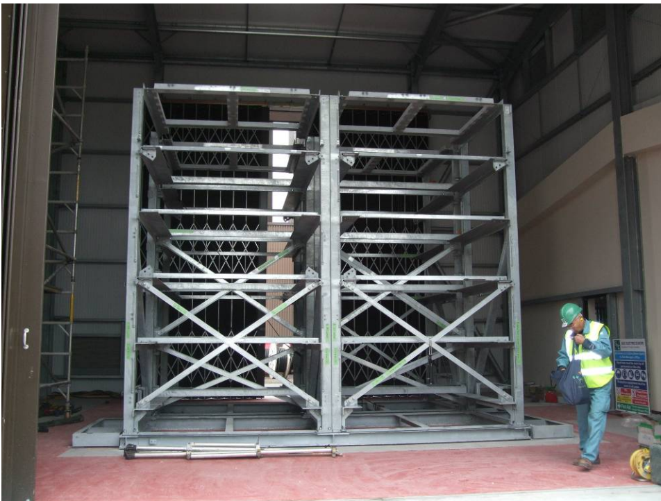
Figure 11 - Installed battery enclosure frame
