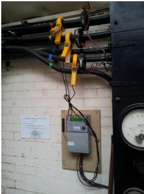
Figure 8 - Example equipment installed in Meadows Crescent East and Lindbridge road distribution substations
