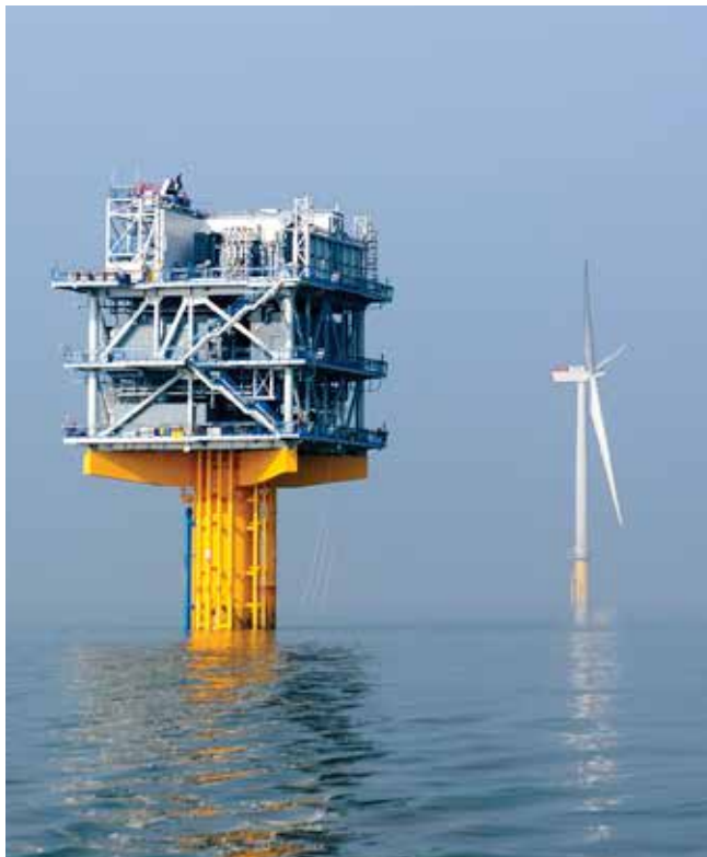
- London Array Offshore substation. London Array Limited
