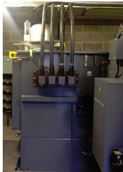
Figure 3 - Transformers with on-load tapchangers
