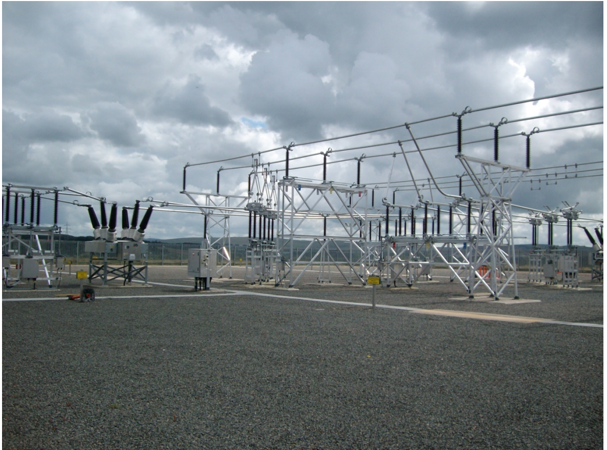
Figure 4.17 –132kV Busbars
