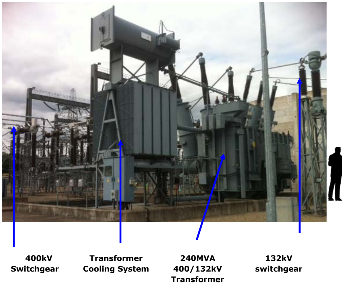
Figure 2. 400kV Substation Bay
