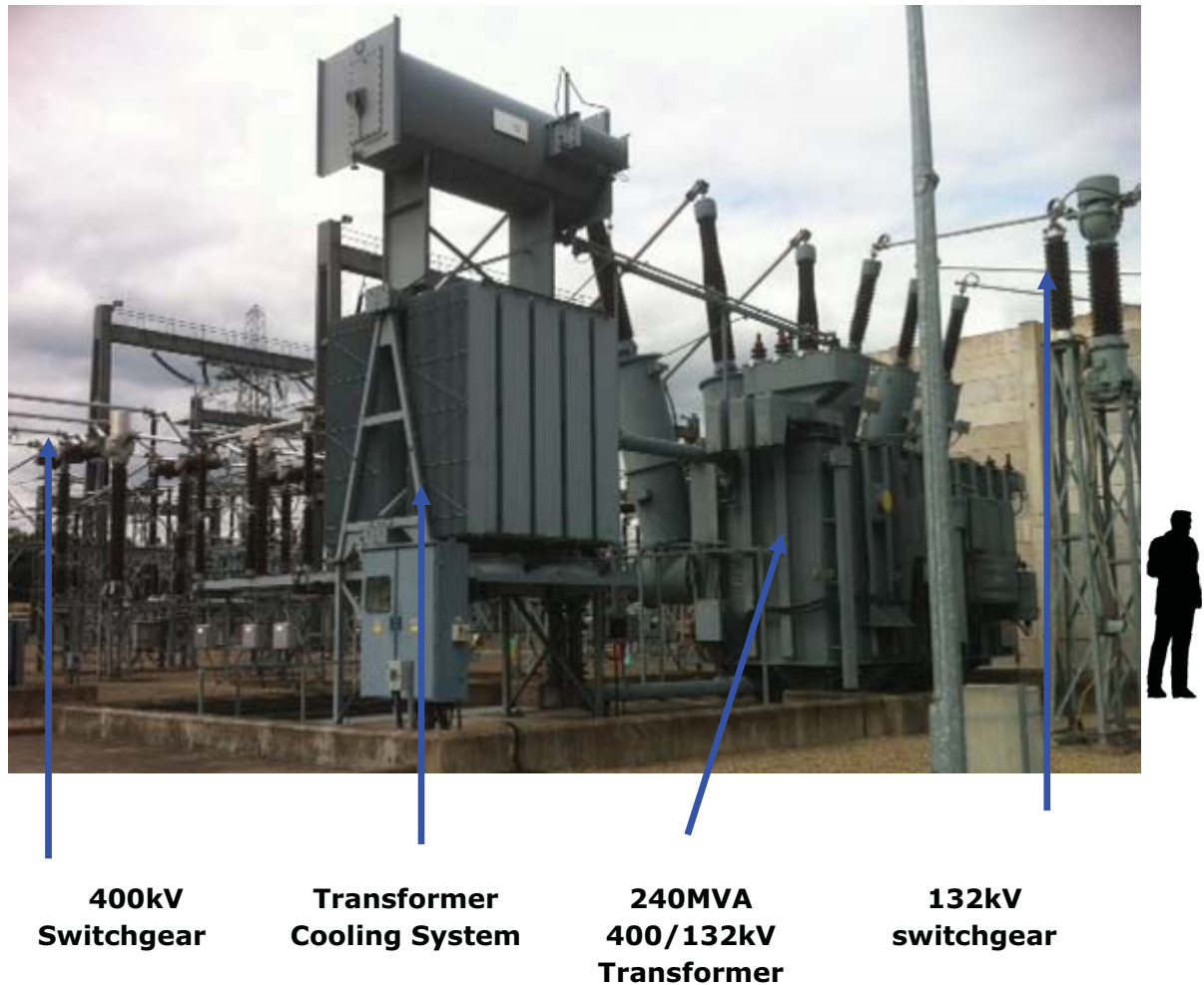
Figure 2. 400kV Substation Bay
