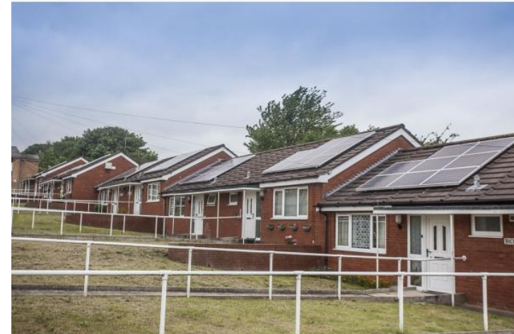
Solar PV on houses in Wrexham
