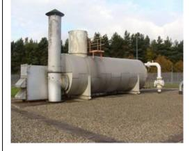
Operation of the units is simple as the burners are usually either 'on' or 'off'. Variances occur where some WBHs have 2 or 3 burners and some burners have 'high' and 'low' fire. WBHs are usually installed in pairs with one WBH capable of providing sufficient energy to
