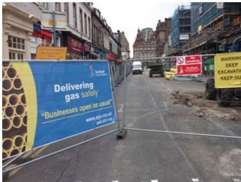
South Queensferry Road, Edinburgh
