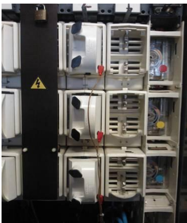
Fuse Carrier with red Auxiliary voltage plugs
