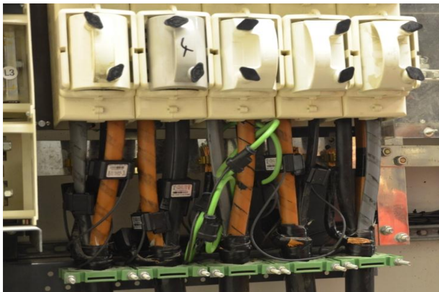
Figure 4: Rigid and flexible Rogowski coil sensors from GridKey. (UKPN)
