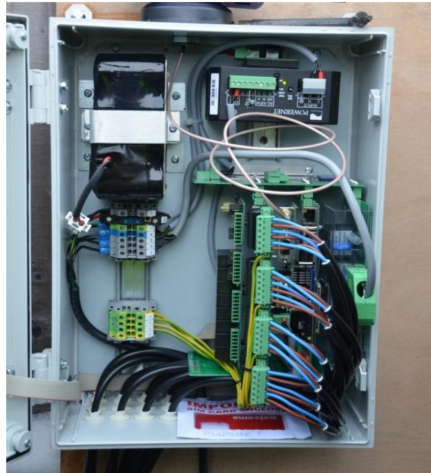
Figures 13: Internal components of the DISCOS I/O metrology unit from PowerSense. (WPD)
