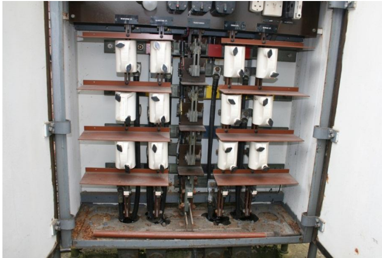
Figure 8: LV Cabinet with open busbar design
