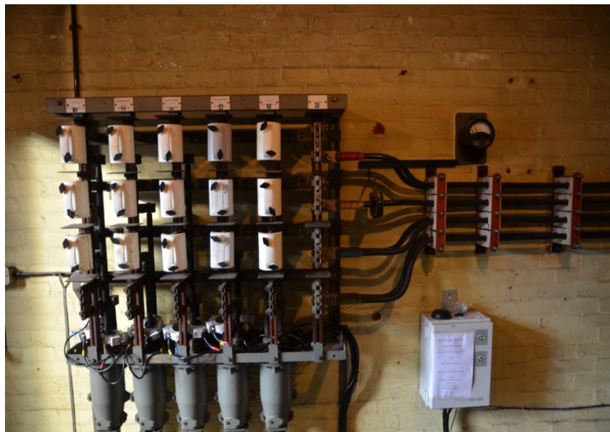
Figure 15: Installation of CTs and DISCOS metrology unit from PowerSense. (UKPN)
