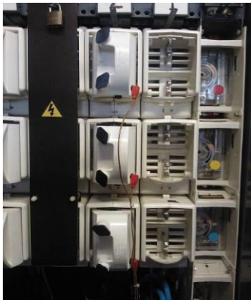
Fuse Carrier with red Auxiliary voltage plugs
