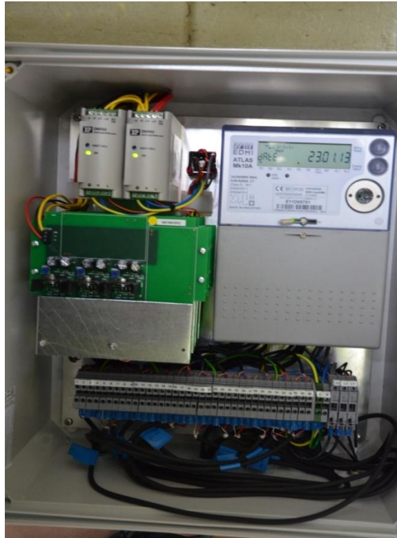
Figure 22: Data aggregation electronic boards and EDM I Atlas Mk10A meter inside the Haysys metrology unit.
