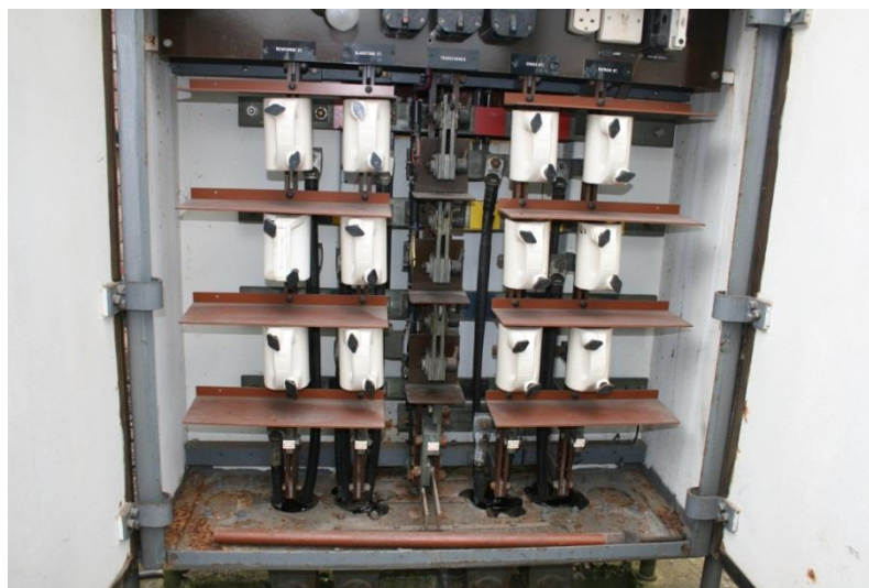
Figure 8: LV Cabinet with open busbar design
