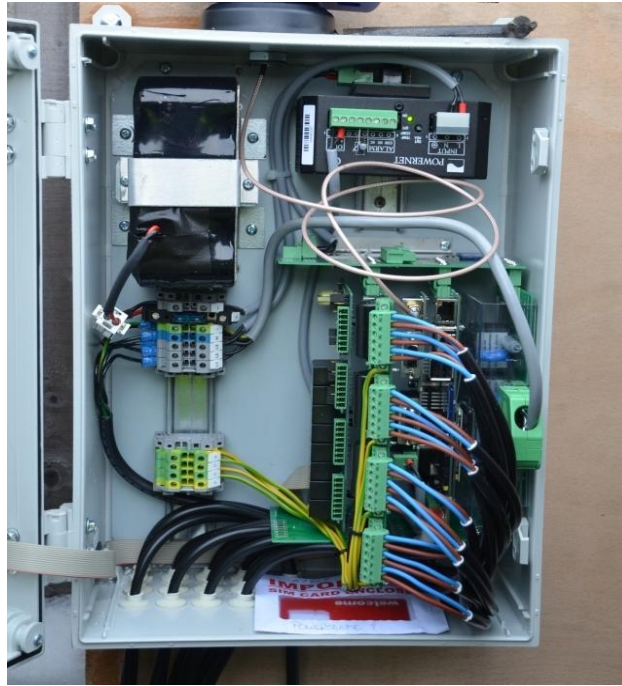
Figure 13: Internal components of the DISCOS I/O metrology unit from PowerSense. (WPD)
