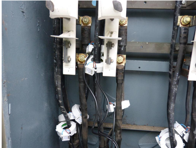
Figures 14: Example of CT installation high up cables due to spacing restrictions. (WPD)
