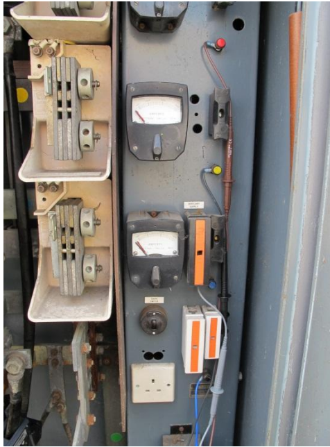
Figure 8: Voltage take off points and fused leads. (WPD)
