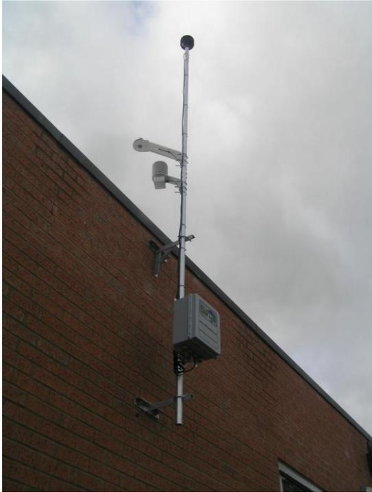
Figure 4-10: Substation-based weather station
