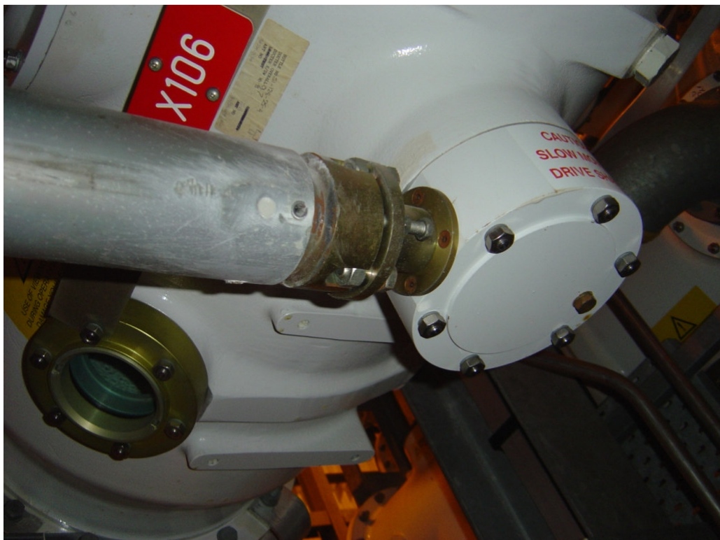
Indoor drive linkage at Sizewell substation
