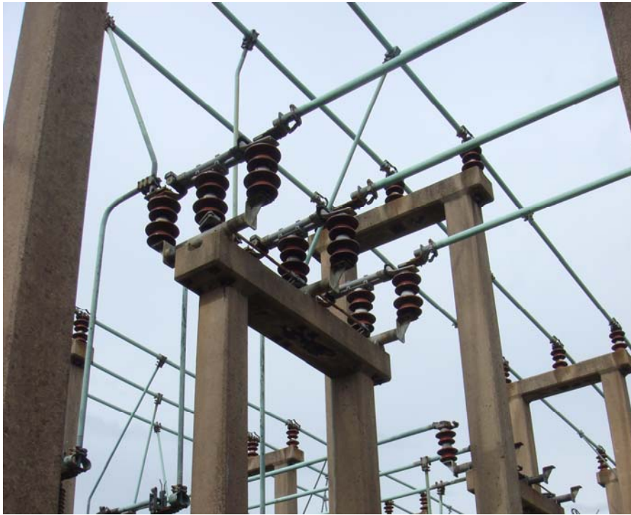
Photograph 3 – View of an undamaged isolator of the same type
