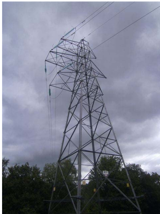
Photograph 2 – Showing the construction of tower 10
